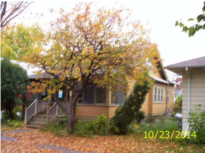
West and south sides, postings
