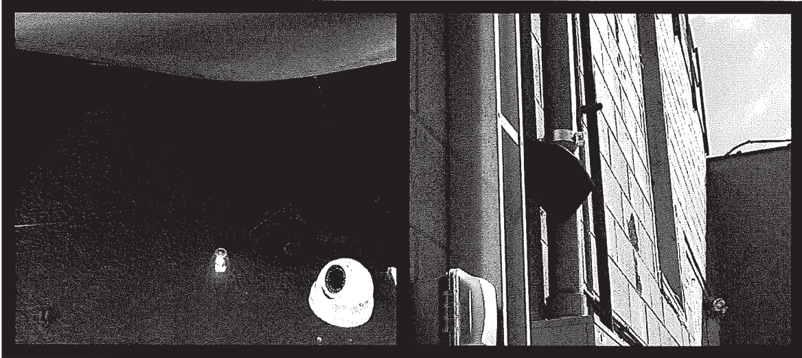
Left: One of two outdoor speakers mounted up and under the awning in front at 1672 Grand (April 11, 2016); Right: One of two speakers mounted on the rear of 1672 Grand (April 11, 2016)
