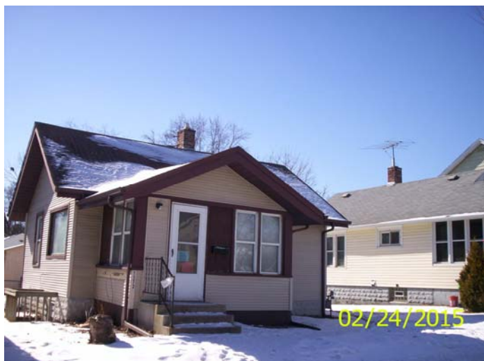
North and east sides, posting
