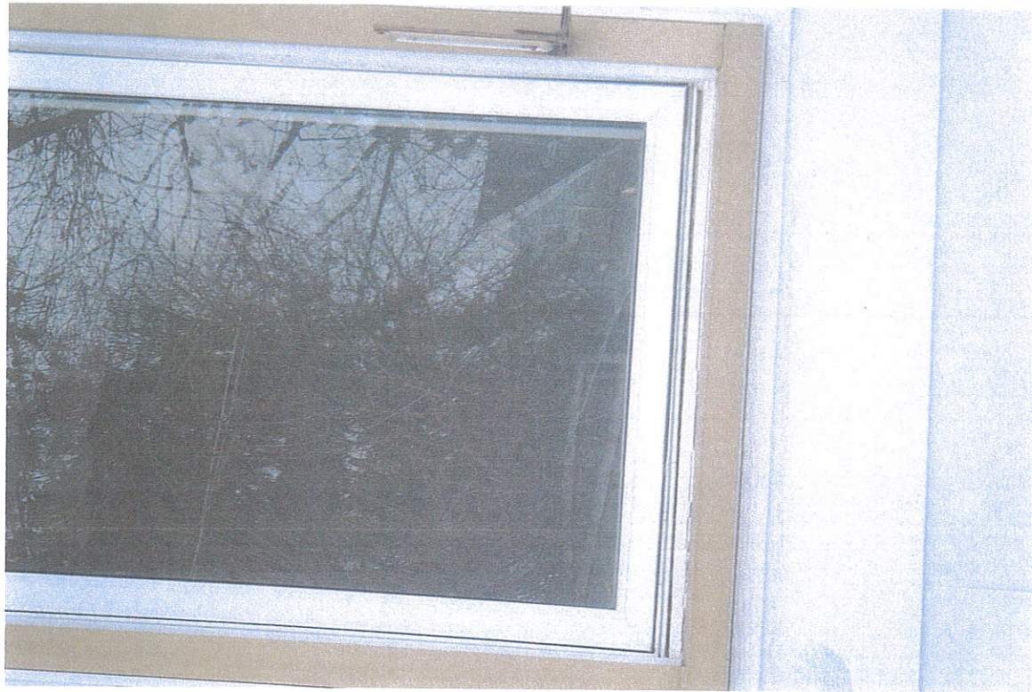
outside window sashes - vinyl clad and frames
