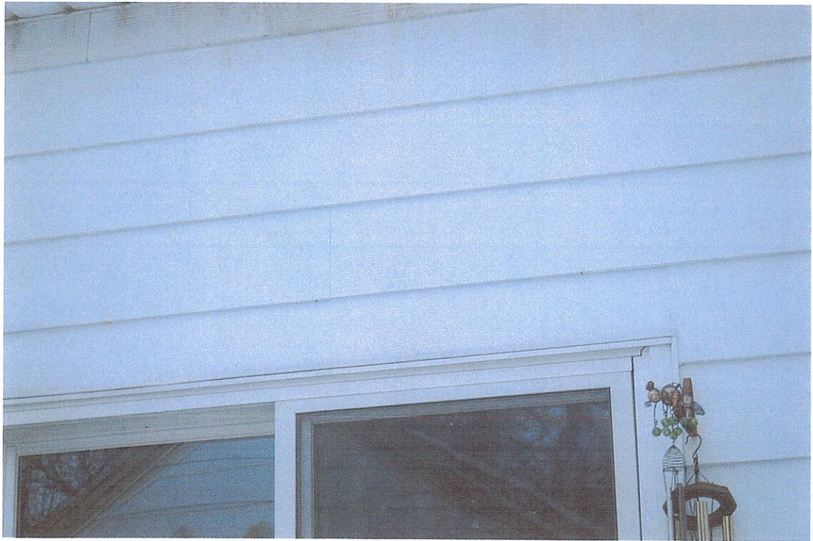
Top of sliding glass door frame
