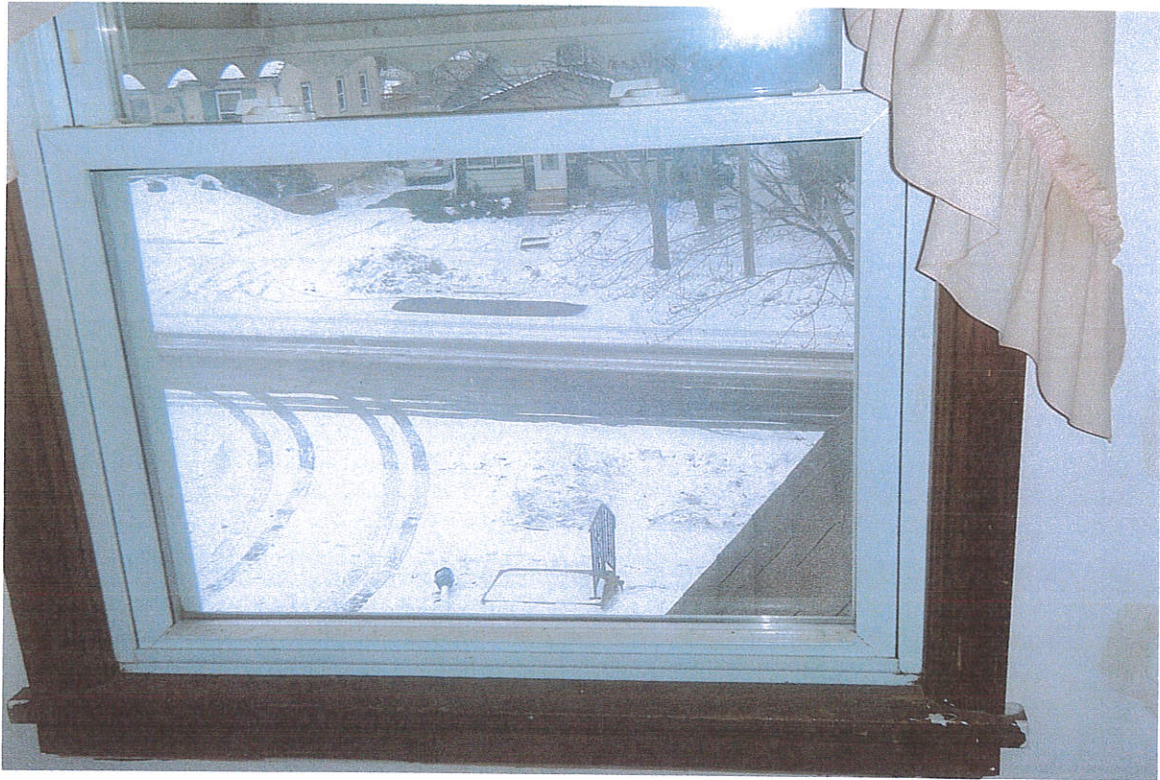
Upstairs Bedroom Windows
