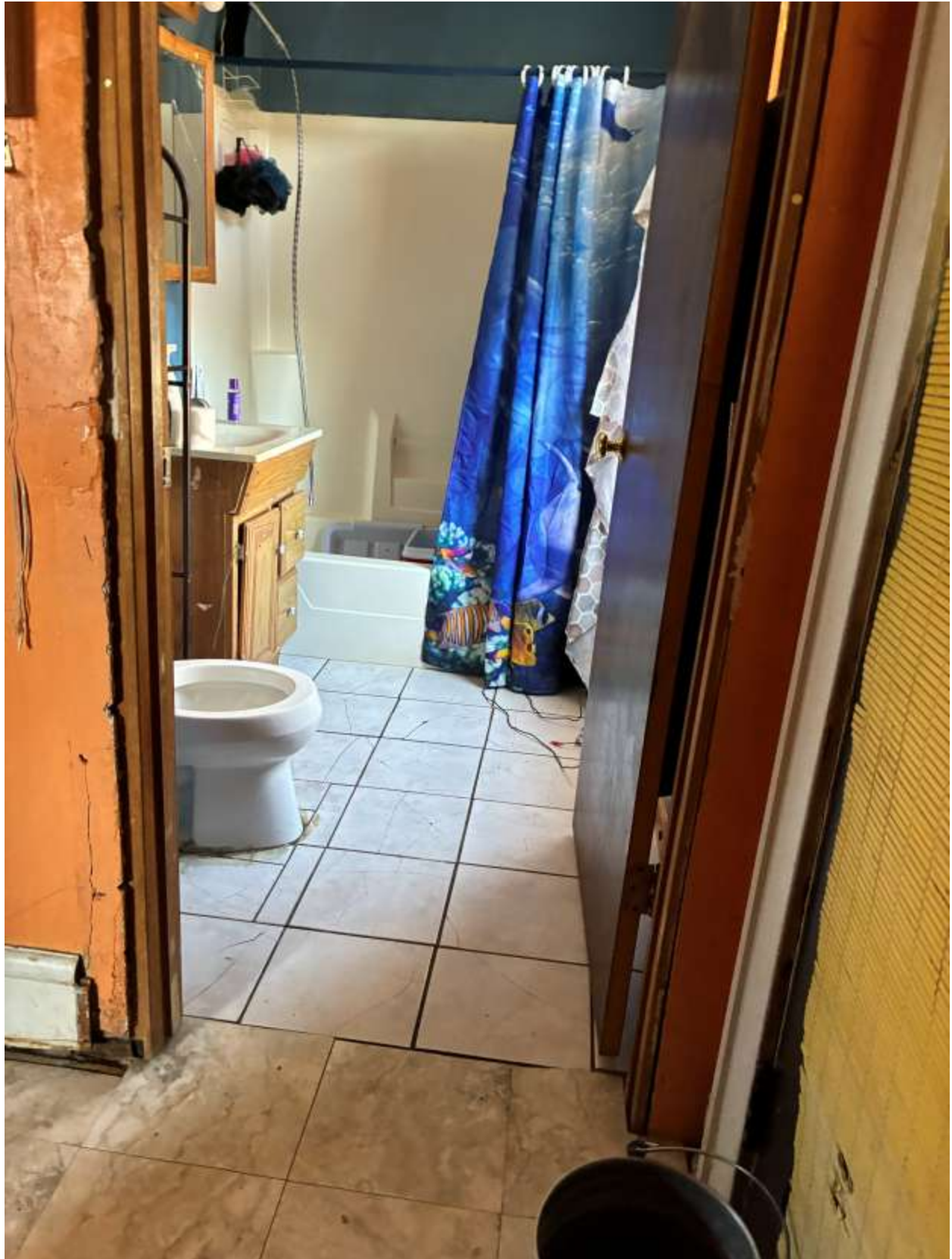
7. bathroom at top of 2nd floor
