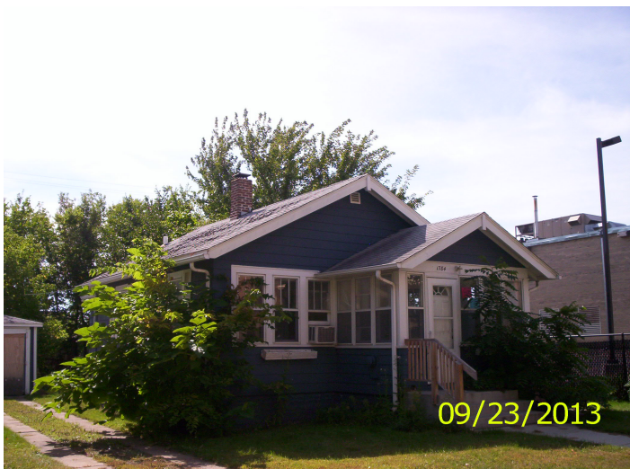
East and north sides, posting
