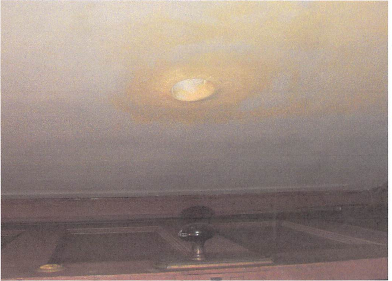
2nd floor wall repaired
