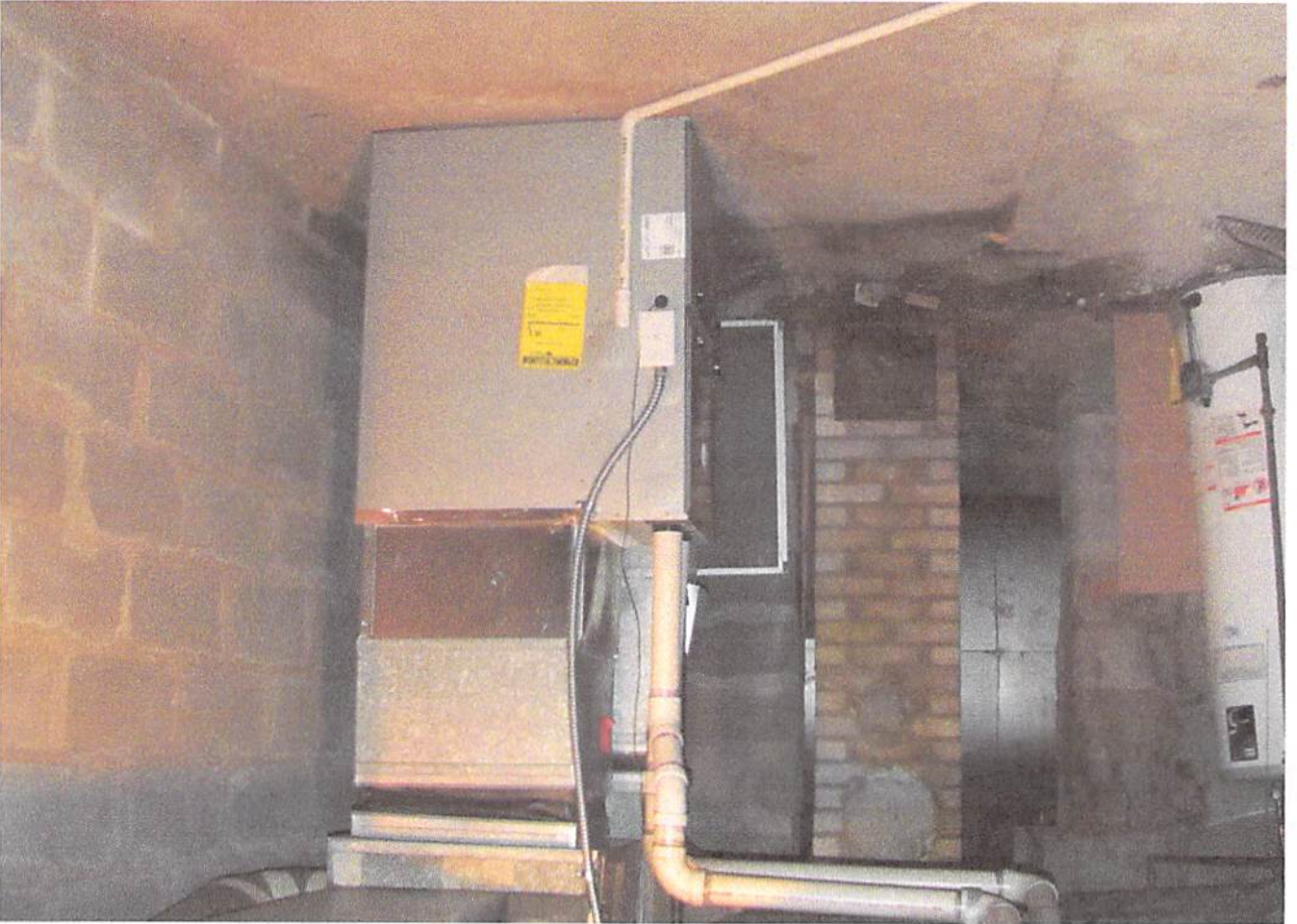
Basement clutter all removed,
