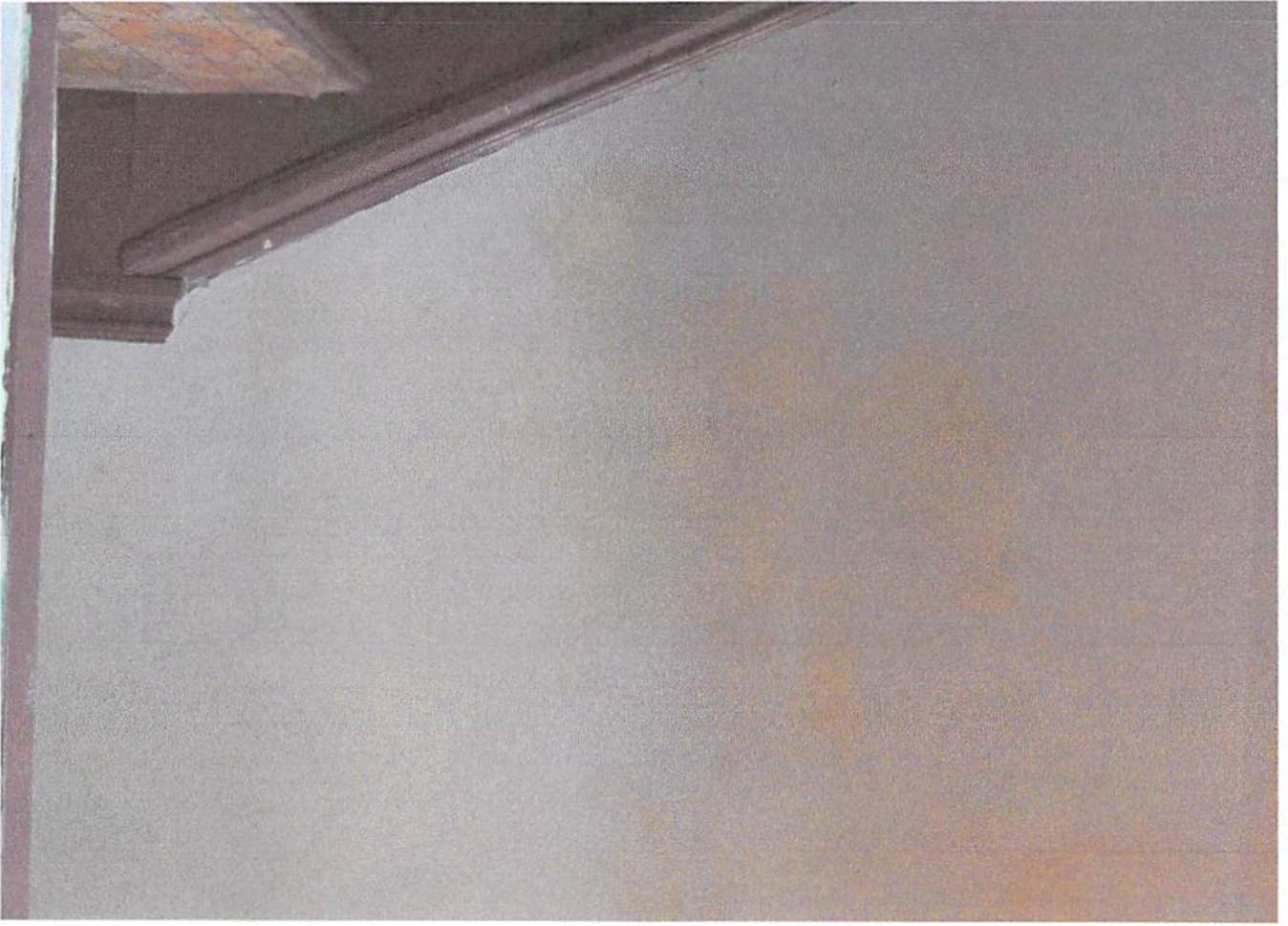
Second floor wall repaired
