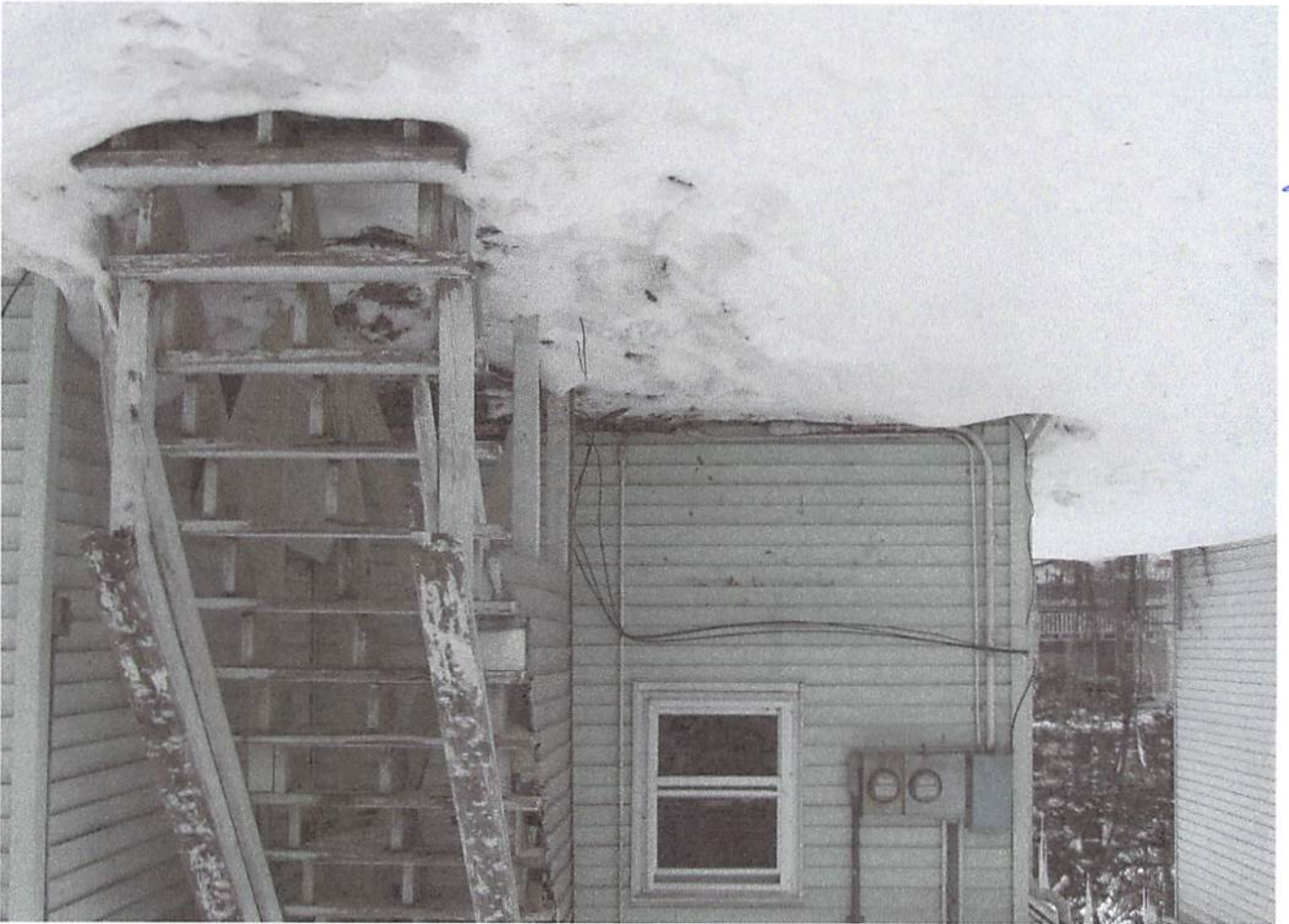
clutter removed by stairs
