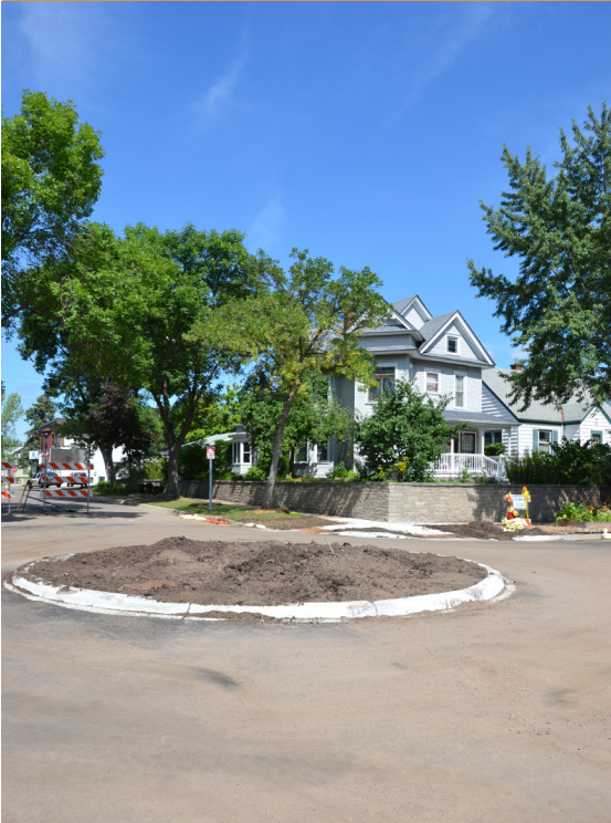
Construction of the Griggs Ave Bicycle Boulevard
