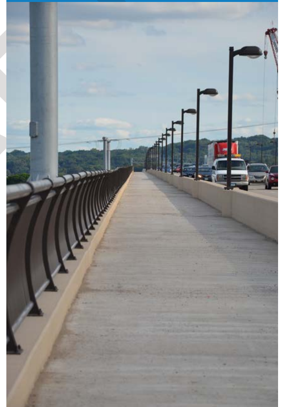
Lafayette Bridge (US Highway 52) over the Mississippi River
