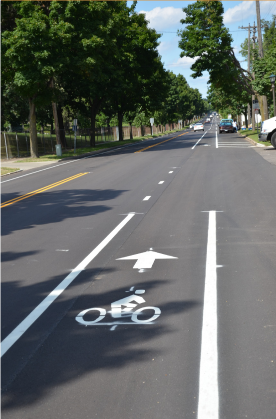
Bike lanes on Jackson St following the mill and overlay process
