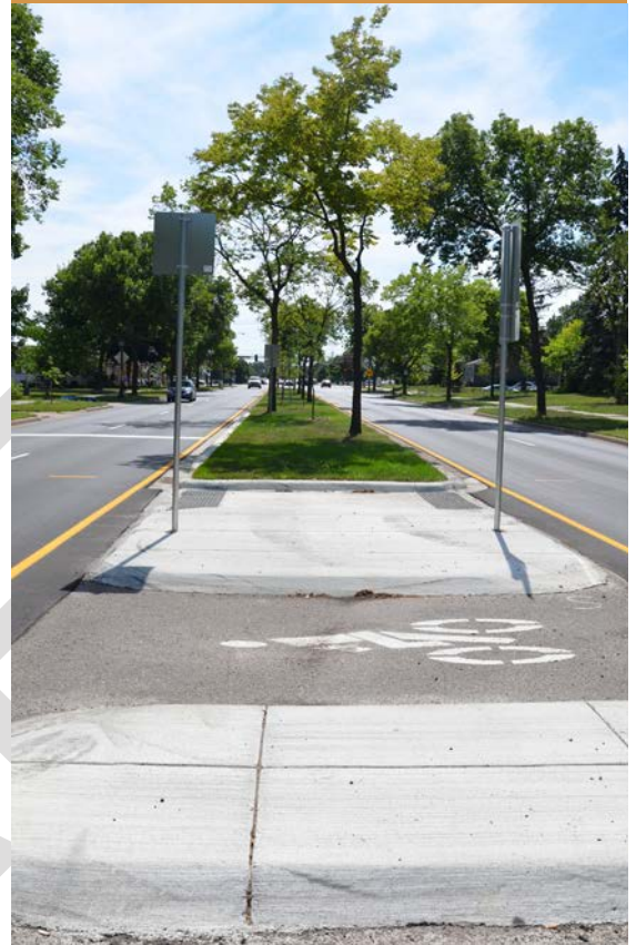
Bicycle and pedestrian refuge islands on Lexington Pkwy aim to minimize conflicts with motor vehicles
