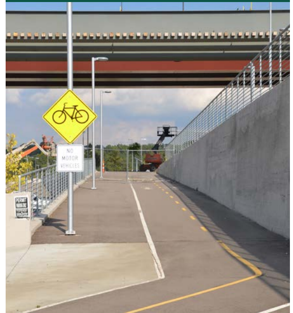
Lighting installed on the under construction Union Depot off-street path
