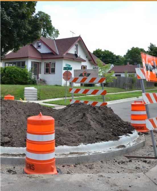
Griggs bicycle boulevard under construction
