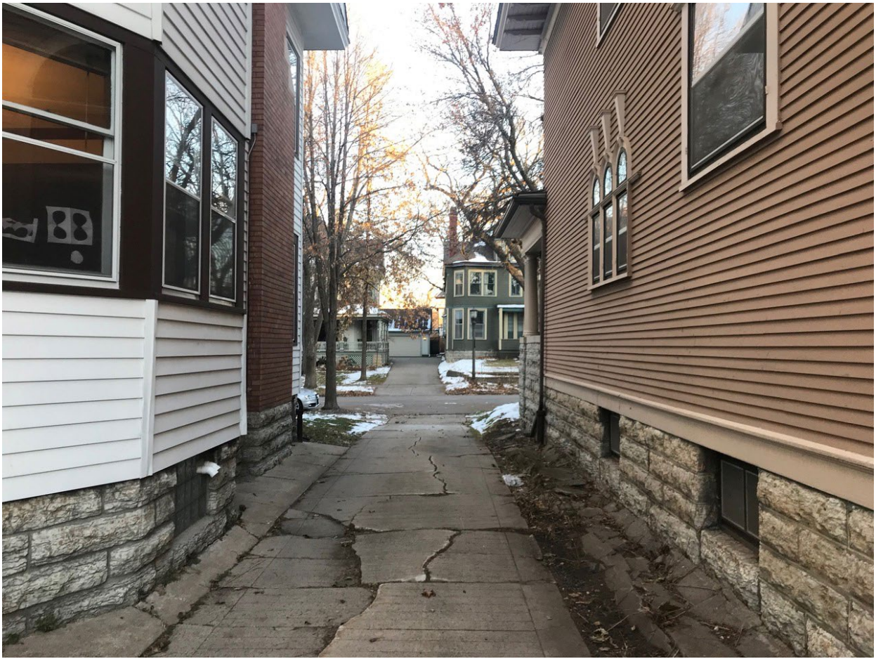
PROPOSED BUILDING SITE (EXISTING TRIPLEX ON RIGHT)
