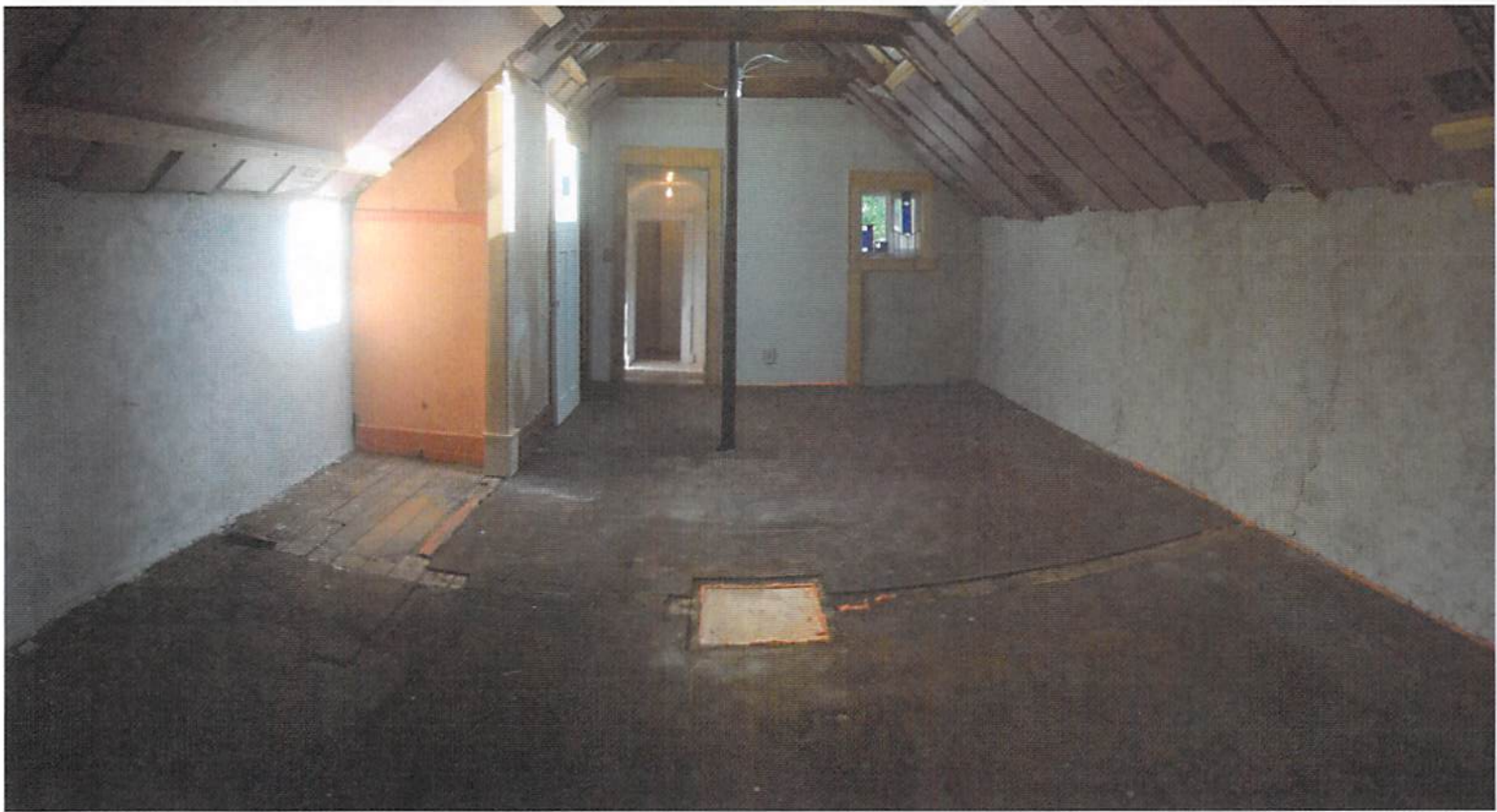
ATTIC MAIN ROOM + ROOM 2 + ROOM3
