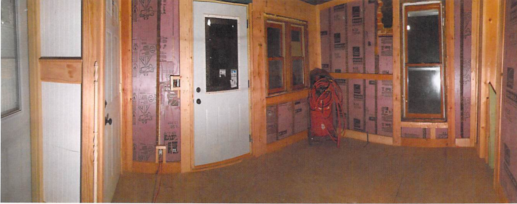
1ST FLOOR BACK PORCH + FRONT ROOM
