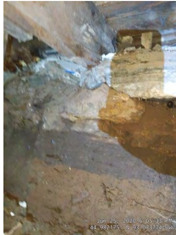
Figure 1: Rotten Joist Ends
