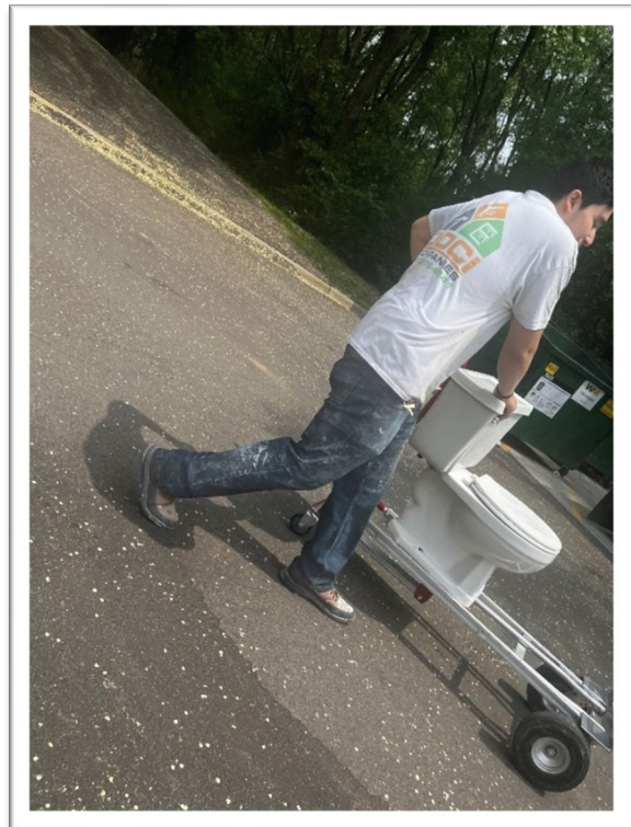
Below: Worker removing toilet.
