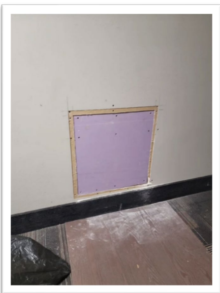
Left: Drywall removal and repair in common area hallway.
