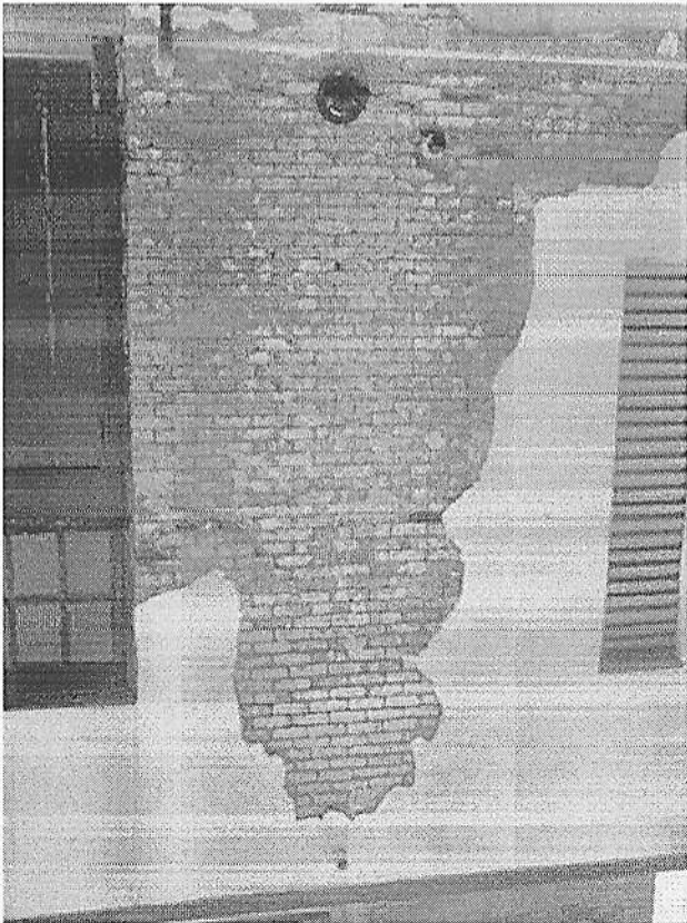
Photograph 3: Scupper —This is a no brainer. Don't dump the roof water onto the wall. This is not an insulation problem. This is just dumb.
