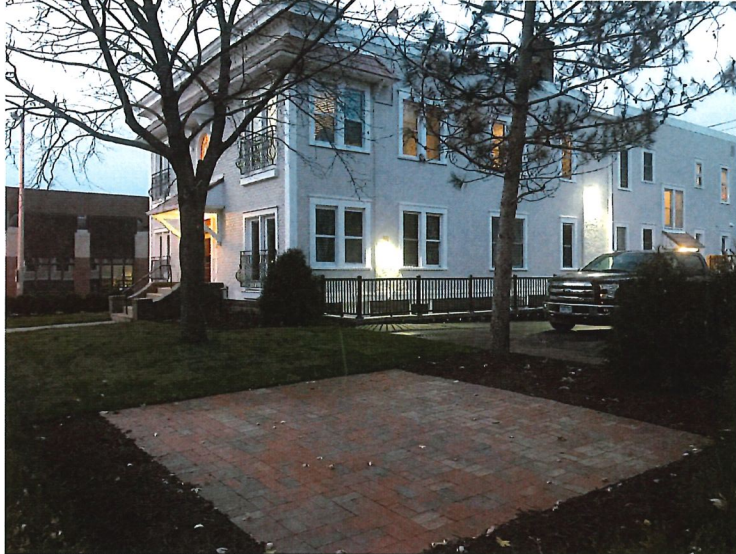
IMAGES: Exterior improvements: new patio and landscaping
