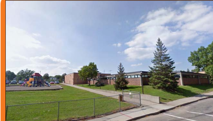
FIGURE 1.10 - Maxfield Elementary , located just east of Victoria Street and north of I-94 is a hub for the local community. The school’s playground represents the only public open space within the station area.
