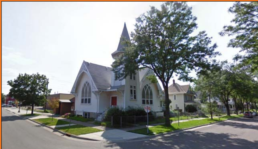
FIGURE 1.8 - The Saint Paul Fellowship Church is a handsome local landmark, immediately visible from the proposed station location.
