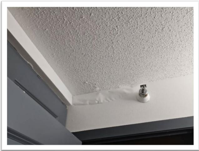
Wall/textured ceiling connection with suspected water damage.
