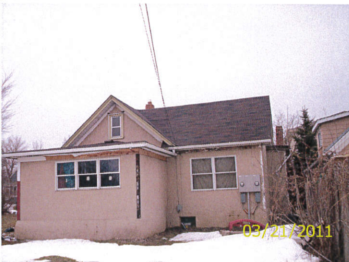
North and west sides of house
