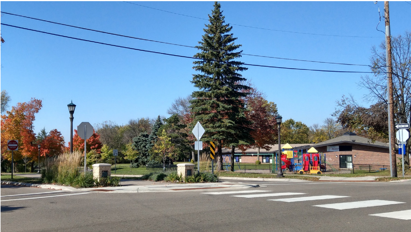
Wheelock Parkway - recently constructed trail crossing at Edgerton Street
