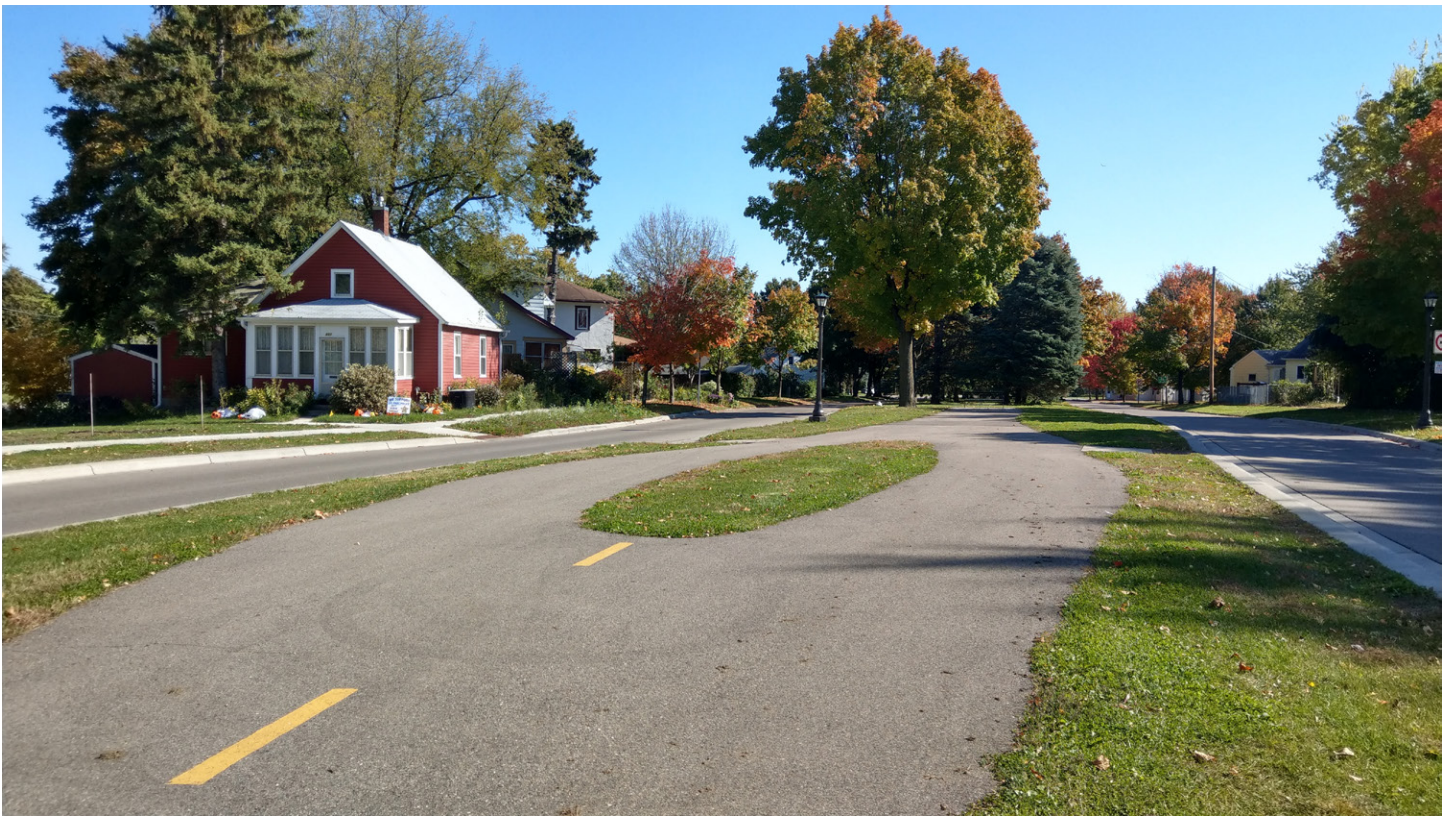
Wheelock Parkway - recently constructed trail section at Edgerton Street
