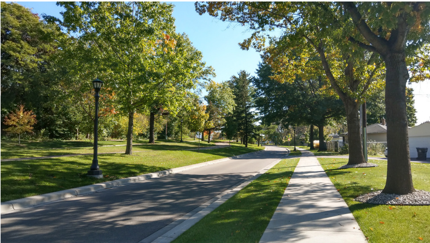
Wheelock Parkway - recently constructed section with trail in the boulevard island
