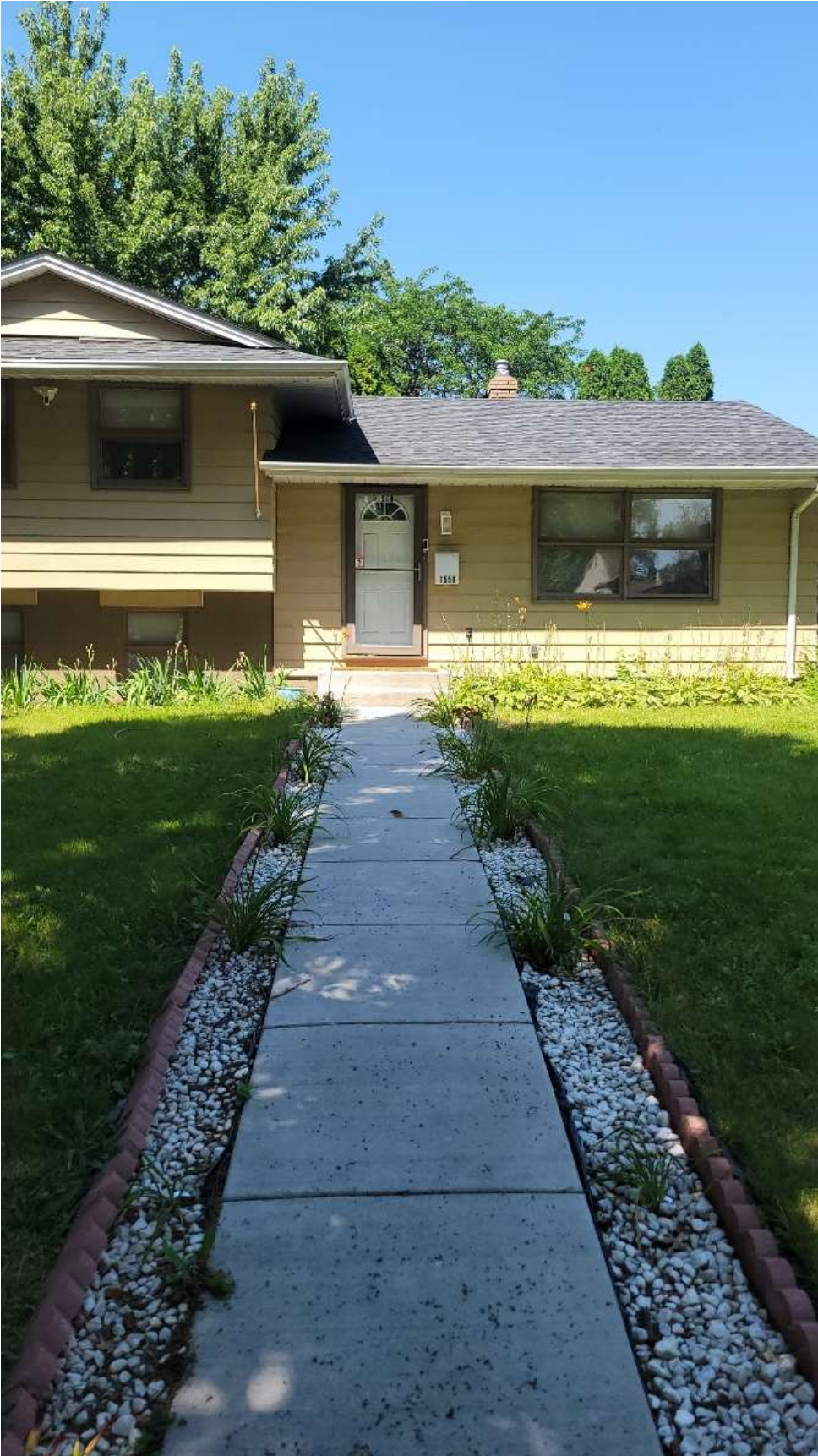
Contractor photos taken 8/2/24
