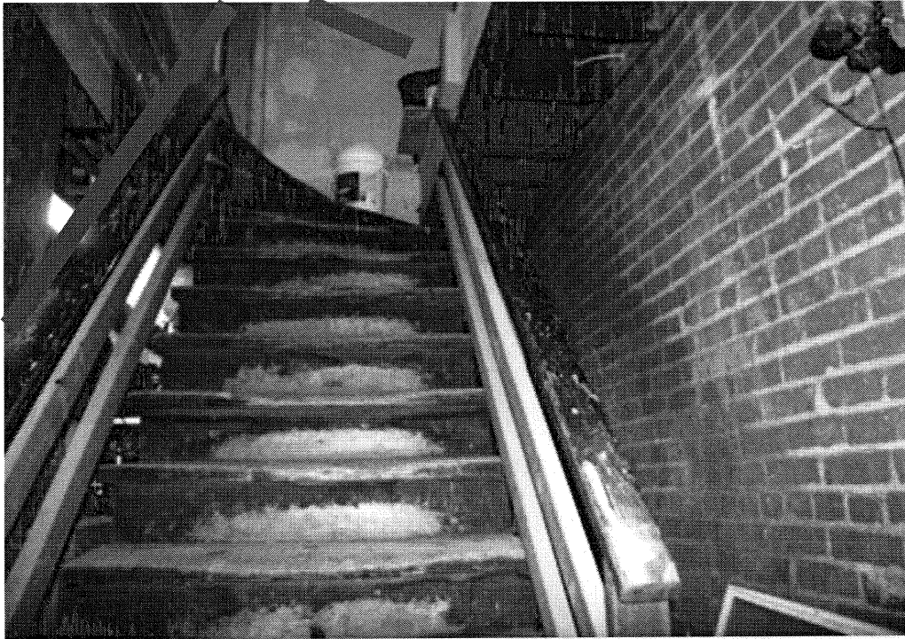
A comfortable hand-rail is to be attached above the two-by-four, thirty-six inches above the stairs.
