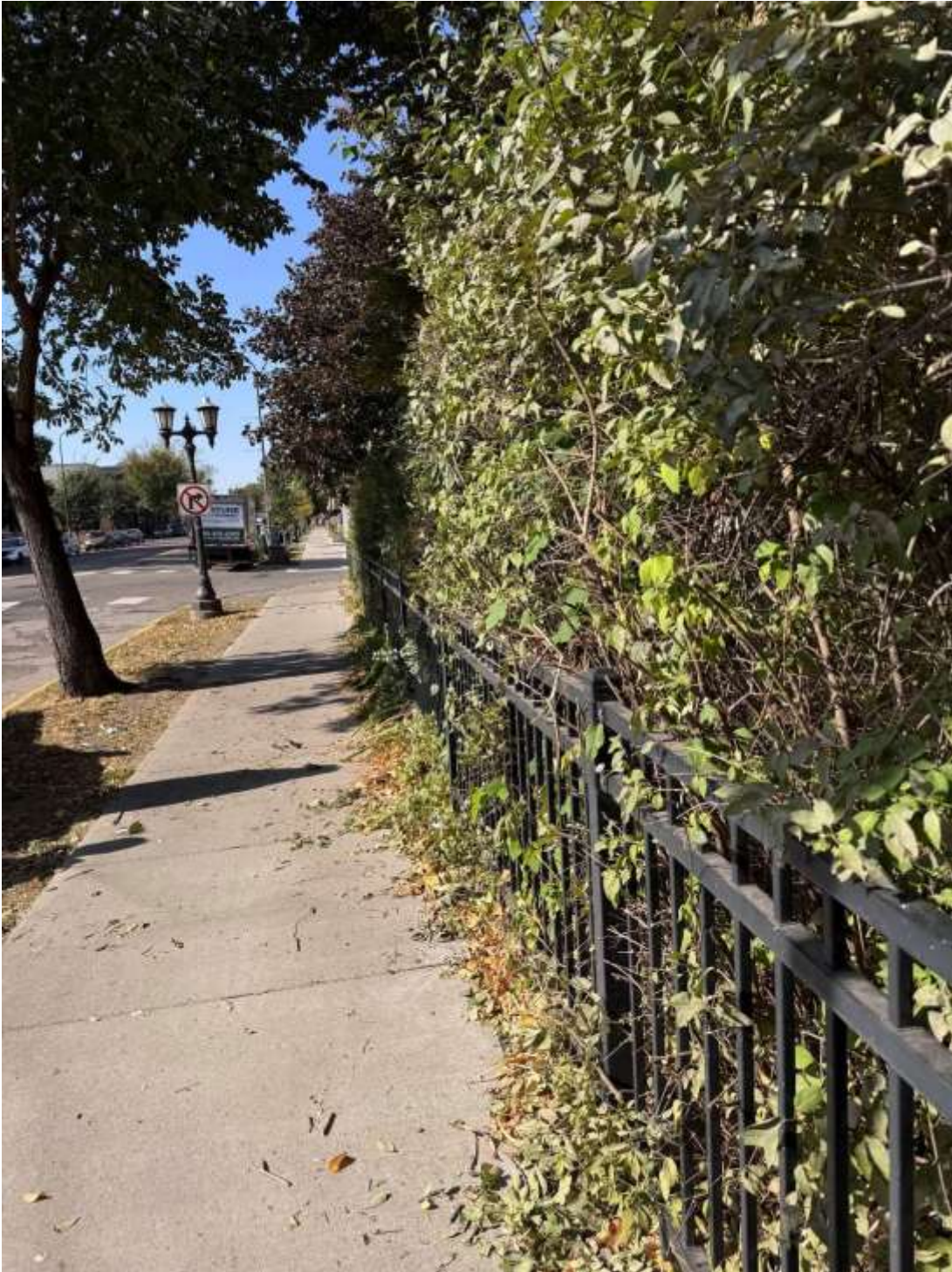
AFTER PHOTO - Grand Avenue side
