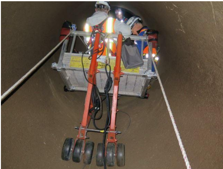
Figure 1 – Winch-Driven Working Stage in 72-Inch Siphon (CUWCD).
