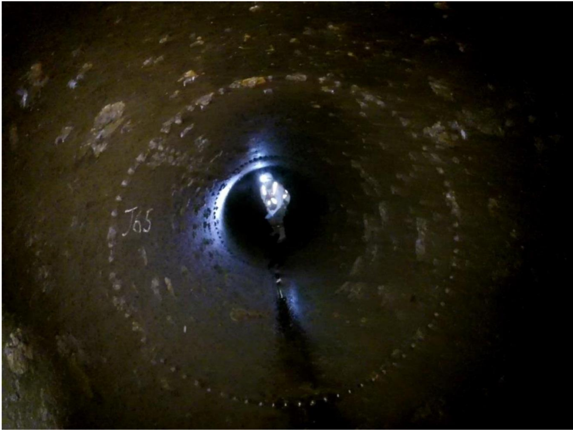
Figure 6: Typical View of Riveted Steel Pipe (RSP).
