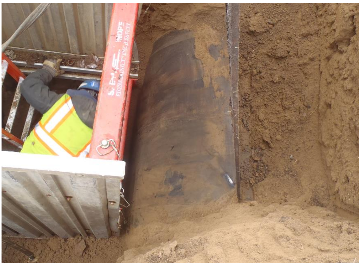
Figure 7: Vadnais Test Pit 4: 1958 V2 steel pipe in good condition.
