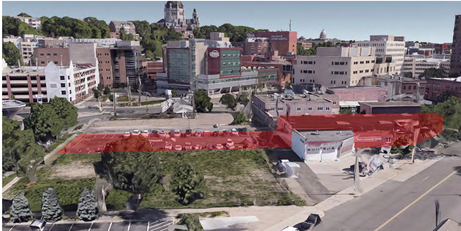
Aerial Photo Looking North
