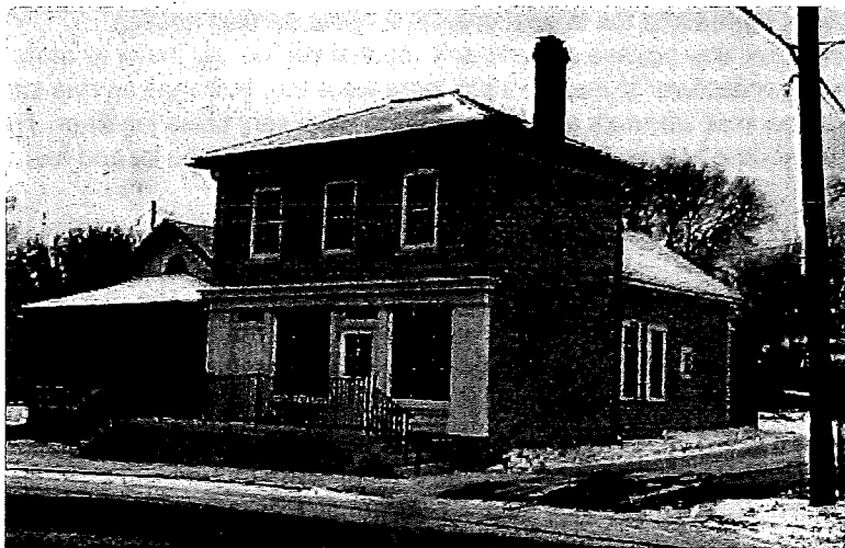
Anthony Waldman House, camera facing southwest.
