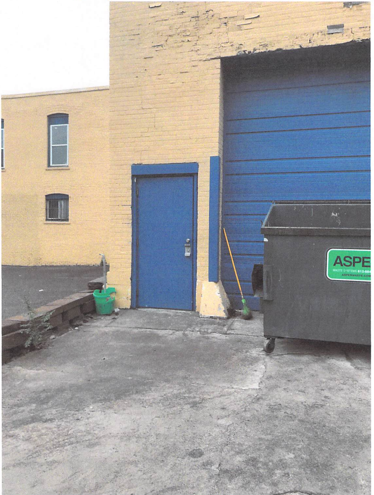
Loading Dock Exit Door
