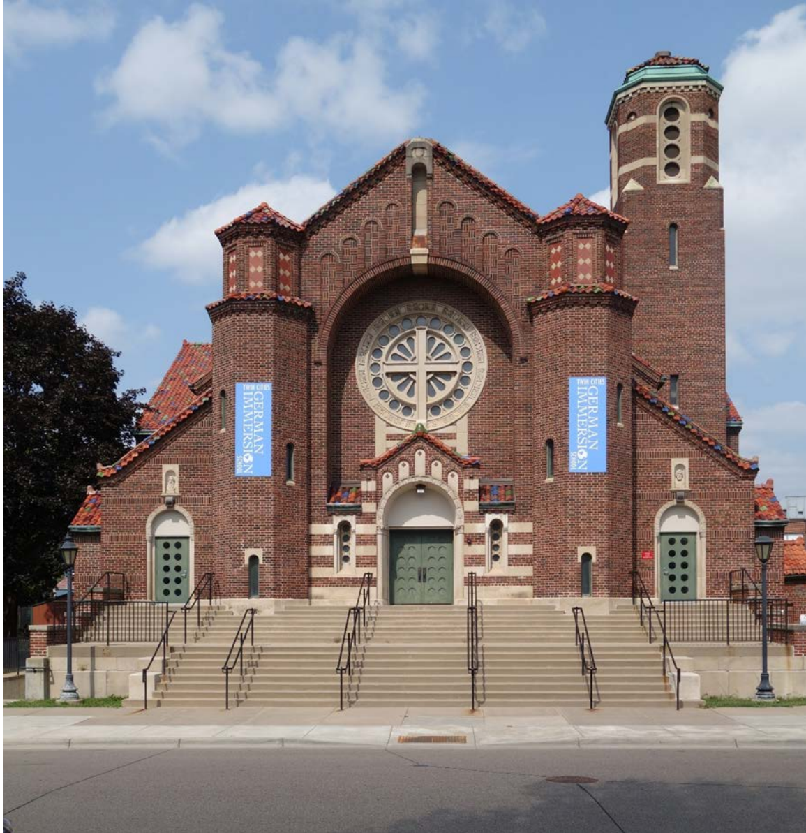
Figure 3. South elevation. Photo Rolf Anderson
