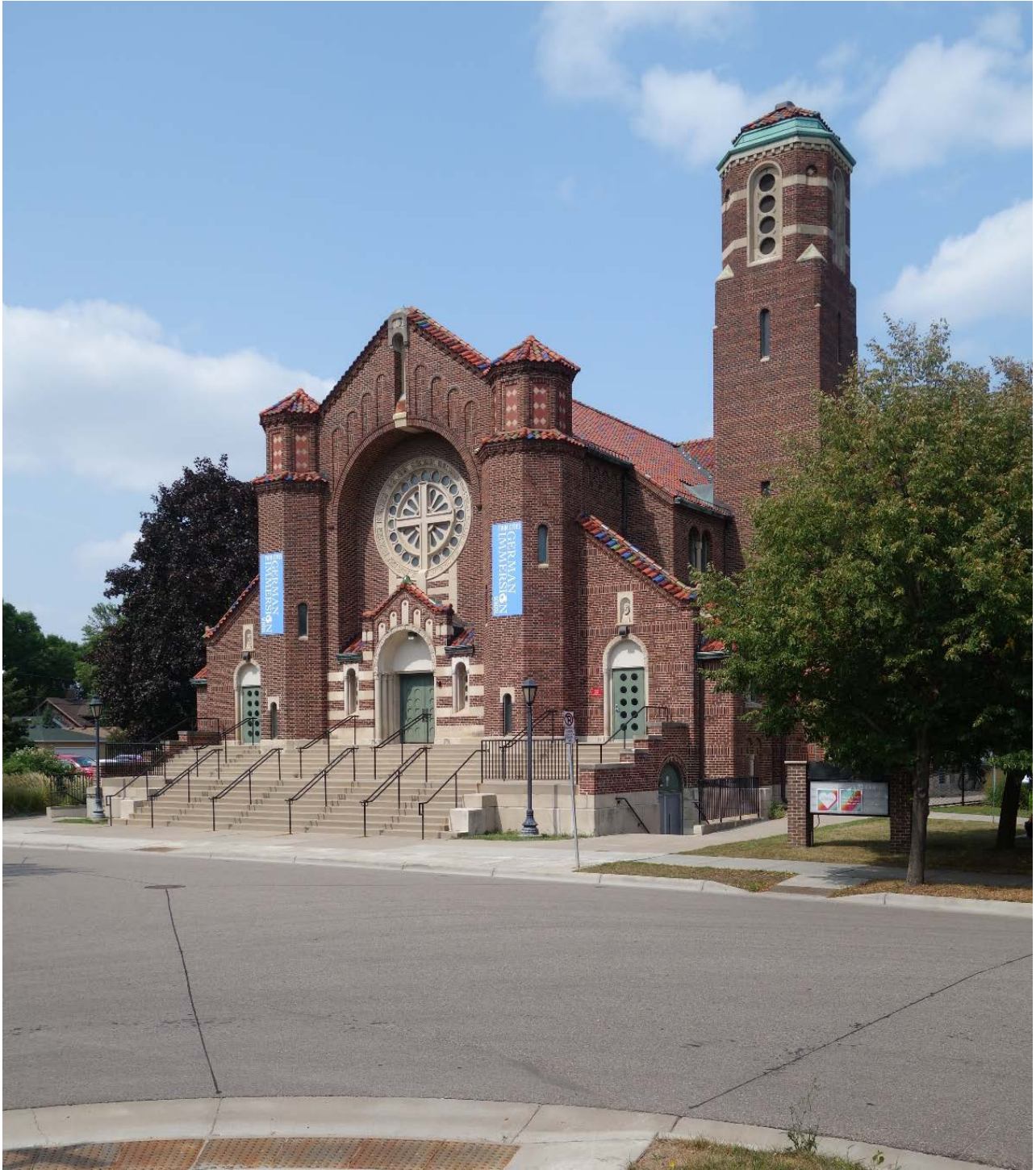
Figure 2. South elevation. Photo Rolf Anderson
