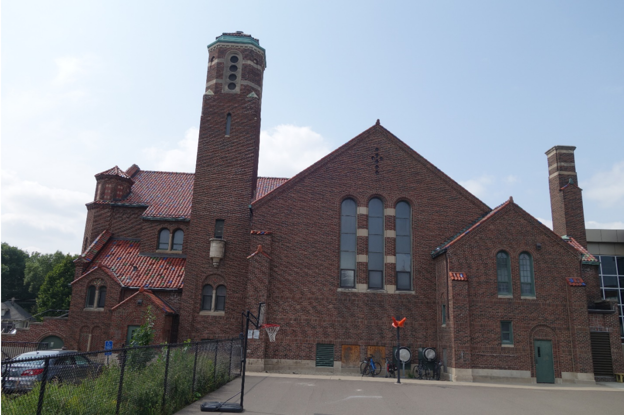
Figure 5. East Elevation. Photo Rolf Anderson
