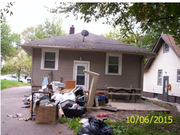
Pile of debris
