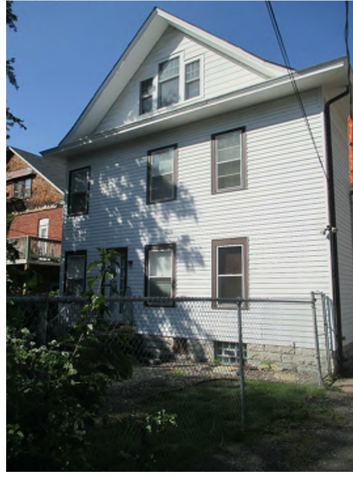
VIEW 12: EXISTING TRIPLEX
