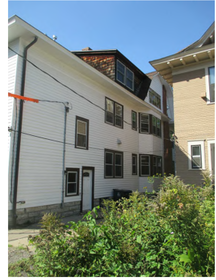
VIEW 14: EXISTING TRIPLEX
