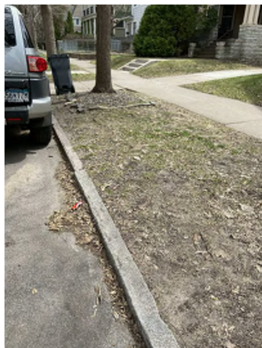
VIEW 05: EXISTING CURB
