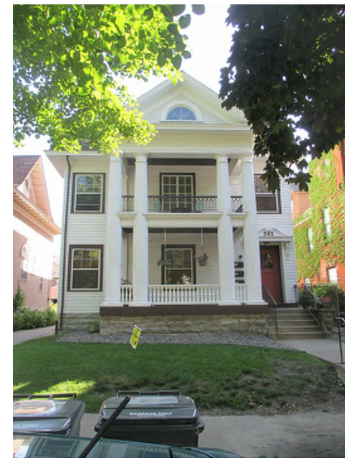
VIEW 10: EXISTING TRIPLEX
