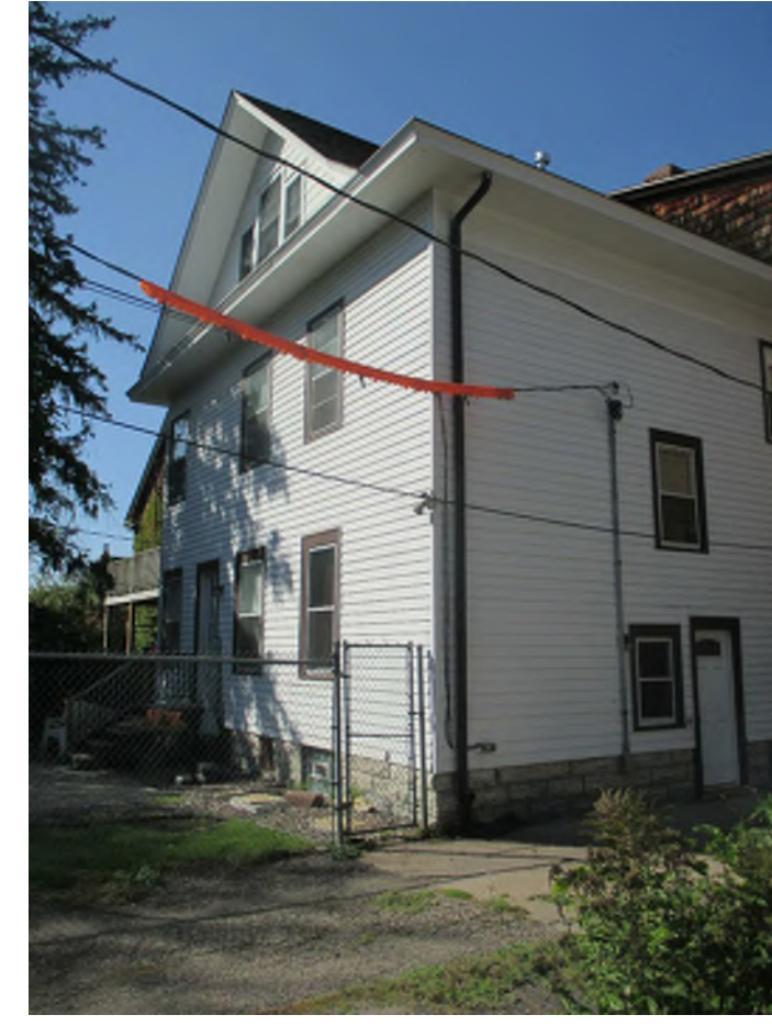
VIEW 13: EXISTING TRIPLEX
