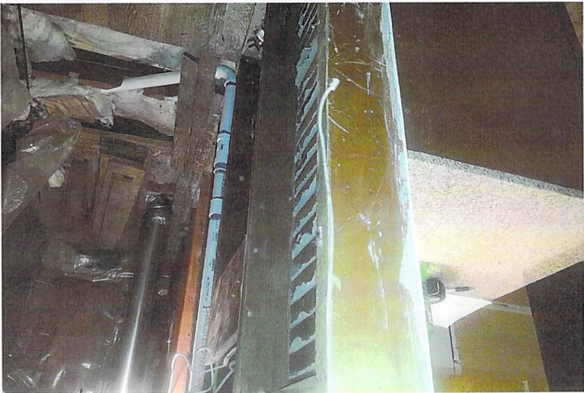
upstairs kitchen remodel 10/14
