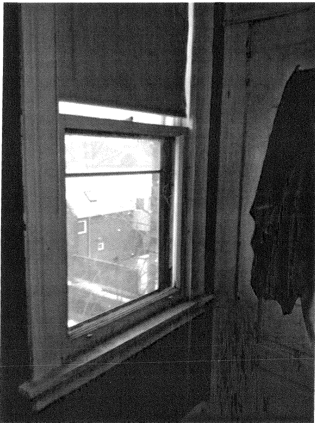
Window located in room
