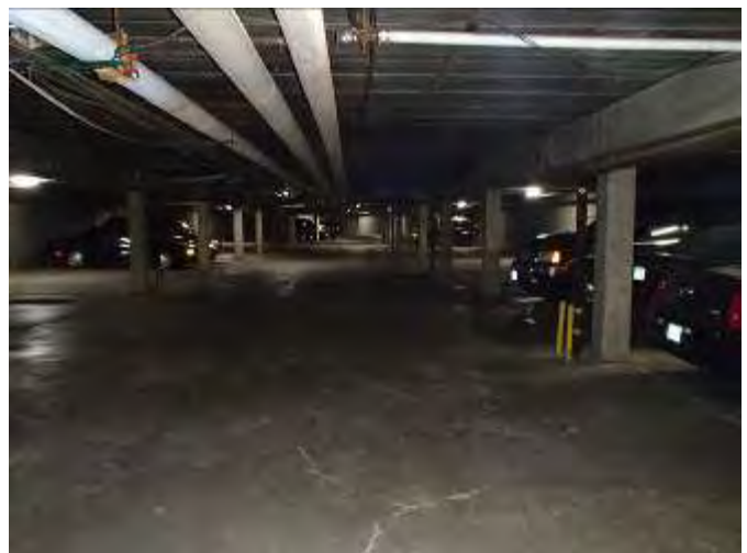
18. Subgrade parking structure for Building 215 (northern and eastern portions)
