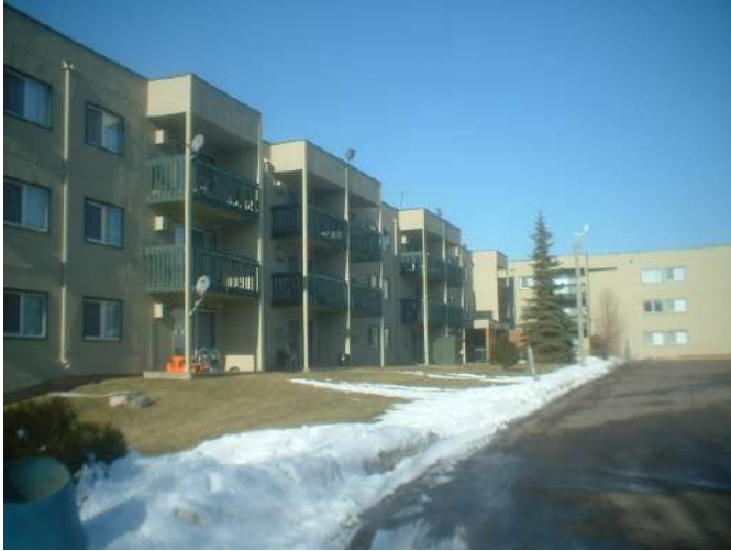
Photo 1 – Typical exterior building elevation
