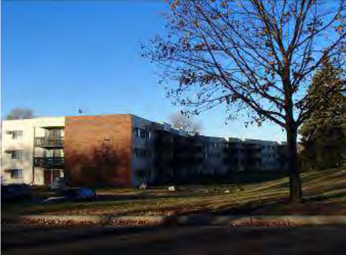
1. Northeast corner and north side of the building, facing west-southwest.
