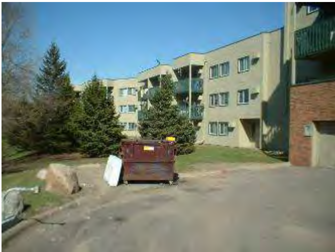
South side of Site building
