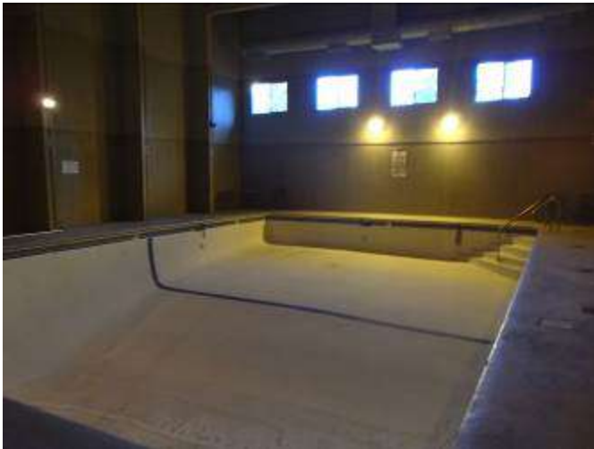
21. Unused indoor pool area.
