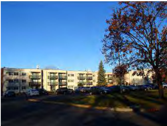
5. East side of the building, facing west-northwest.
