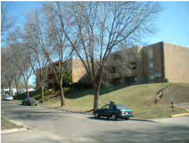
Adjacent property east
