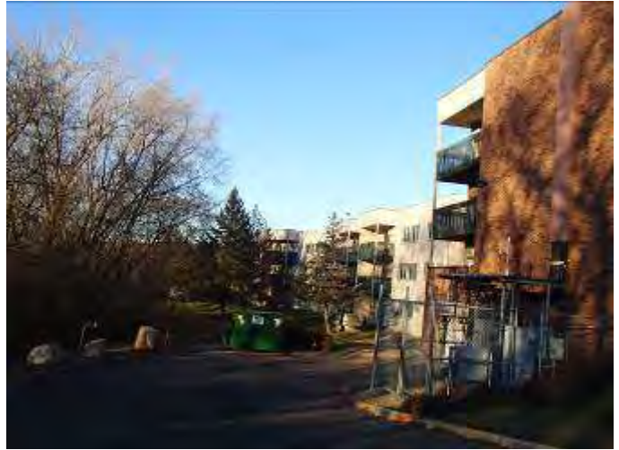
4. South side of the building, facing west.
