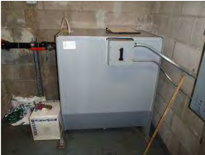
15. Elevator motor for the elevator within the 200 Building, located in the 200 Building garage.
