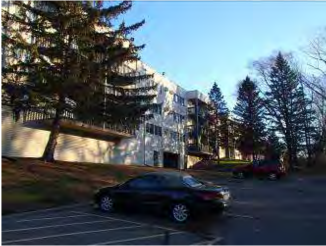
3. South side of the building, facing east-northeast.
