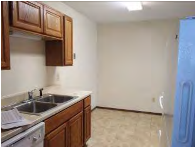
9. Kitchen area in vacant unit
