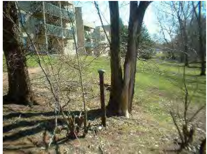
UST vent pipe
