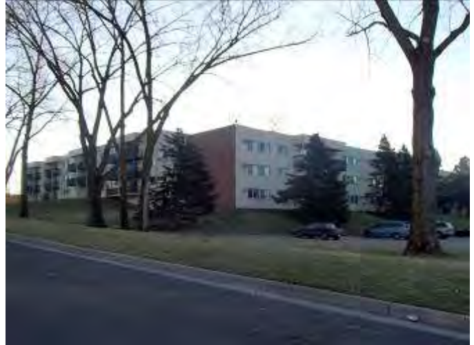
2. North and west sides of the building, facing southeast.
