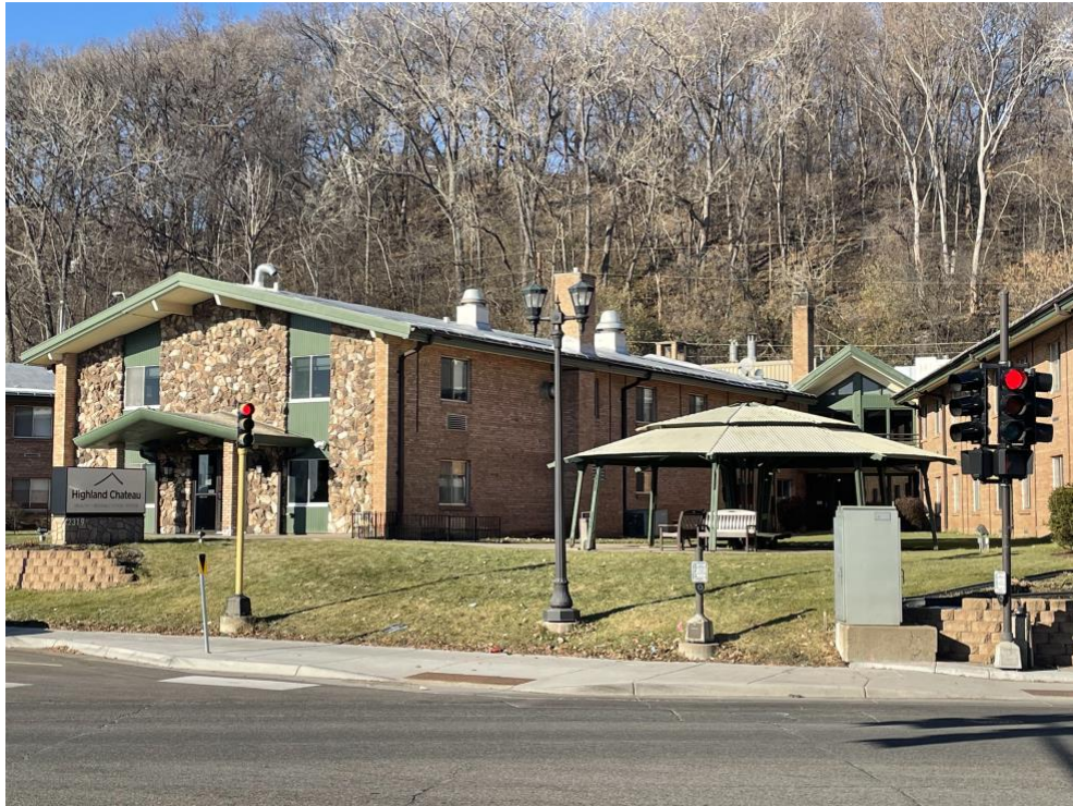
Photo 1- existing Highland Chateau (proposed development behind)
