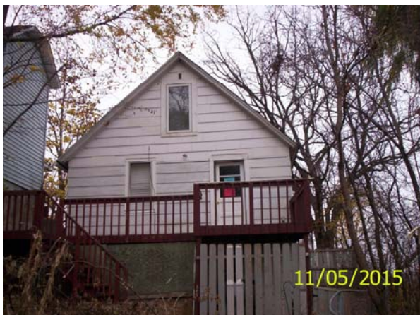
South side, posting
