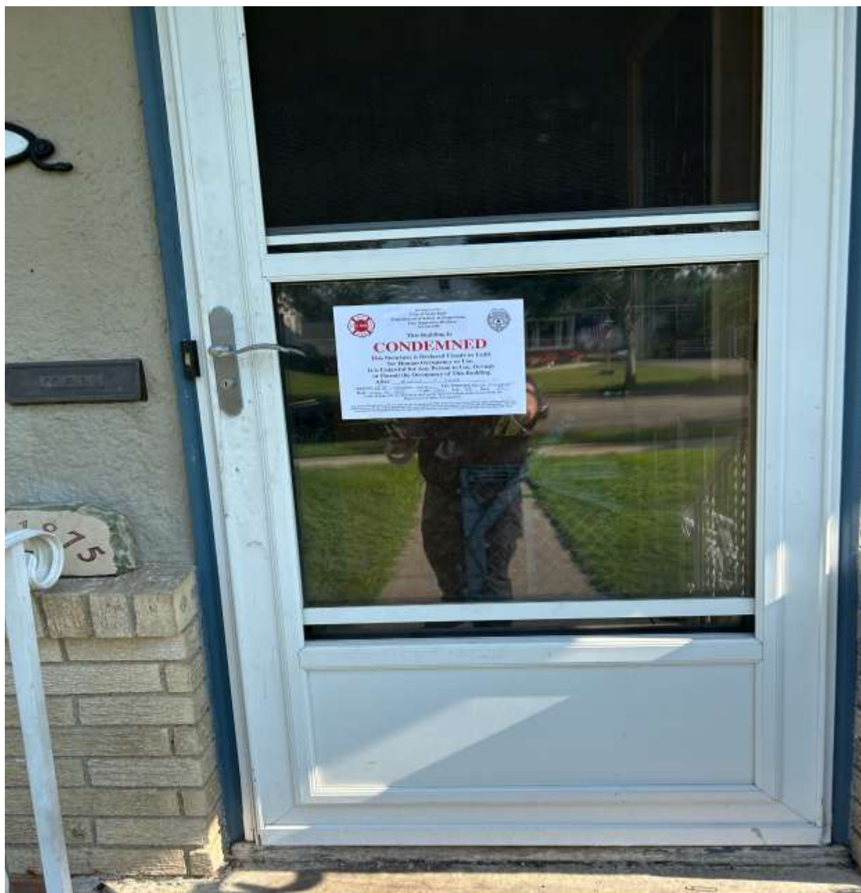
1875 Nebraska Ave E. Condemned placard
