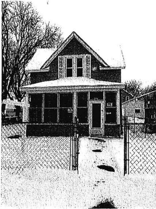
Photo 1 – North Elevation of 956 Geranium Ave
