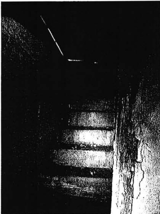
Photo 7 – Stair Access Allowing Moisture Infiltration
