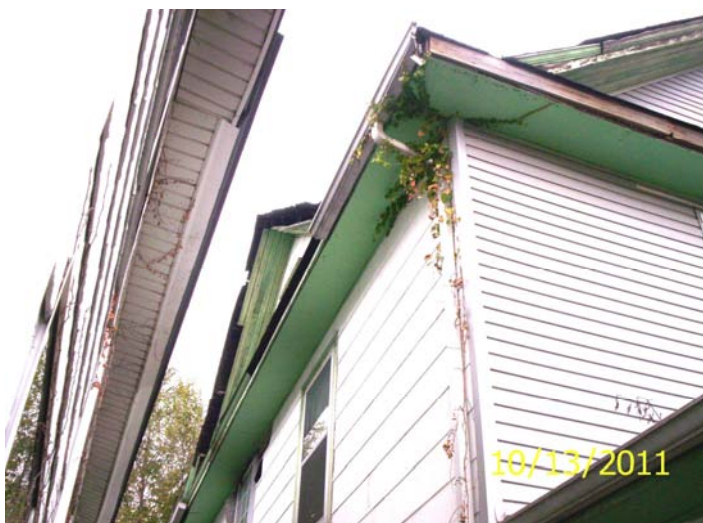
North side eaves
