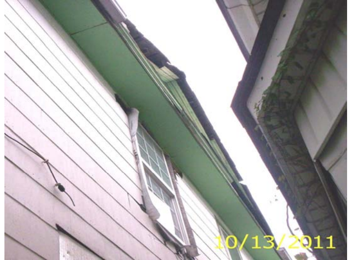
North side eave, unfinished window installation
