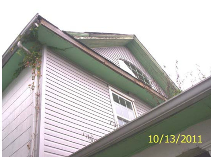
West side eaves
