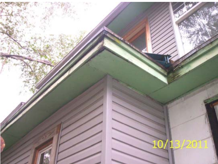
Eave of the east side flat roof
