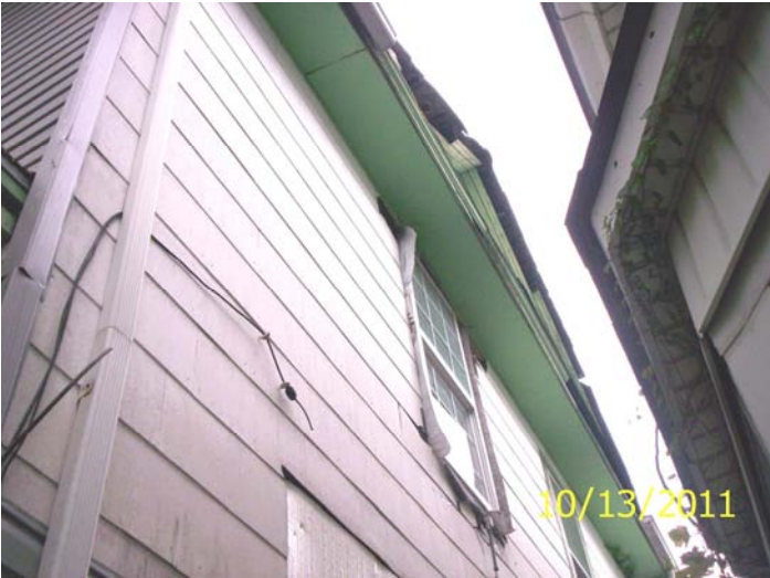
North side eaves
