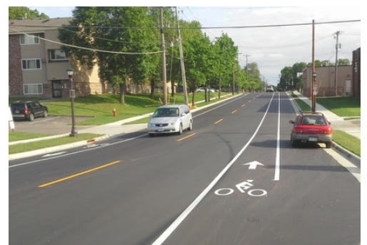
An example of bicycle lanes on Western Ave
