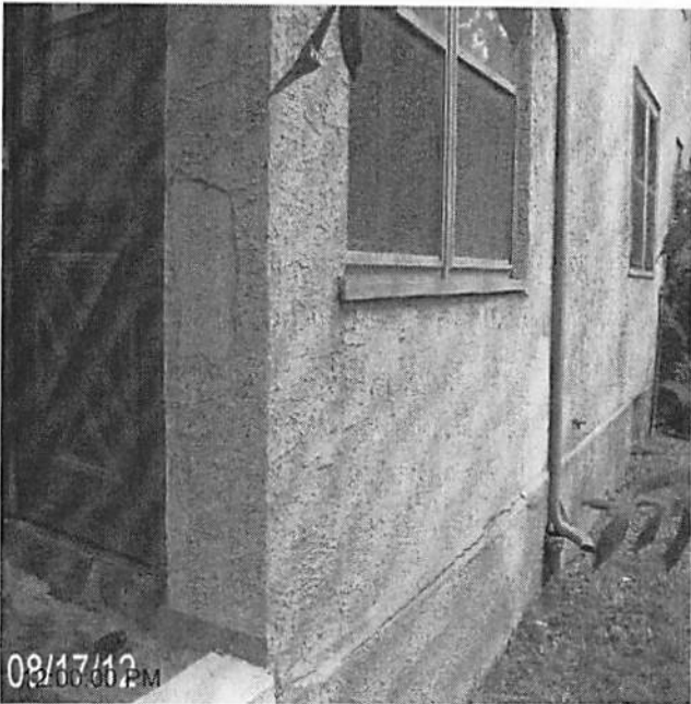
Date Completed: before: repair pressure wash stucco
