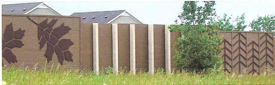
Noise barrier - MnDOT standard concrete post/wood plank
