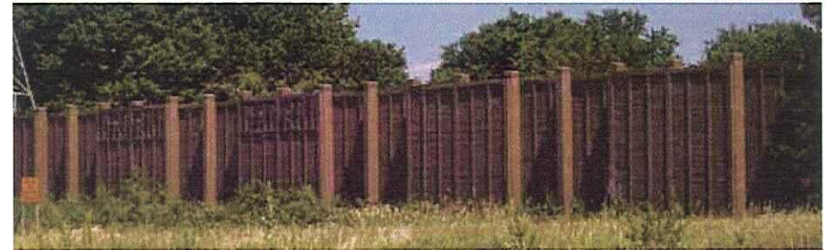
Noise barrier - MnDOT standard concrete post/wood plank
