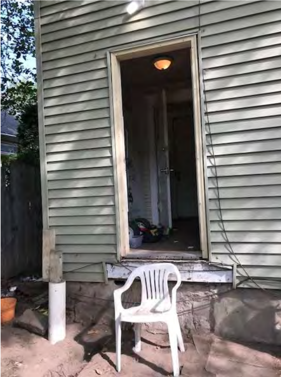
Unit 2 Main Entrance – from the Rear.
