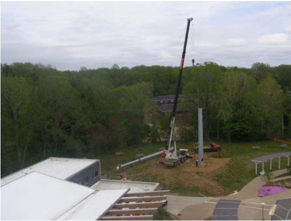
Fig. 2 The tower under construction May 5, 2007
