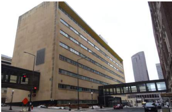
Figure 2.16: Block D, Minnesota Mutual Life Insurance Company/ Pioneer Press Building
