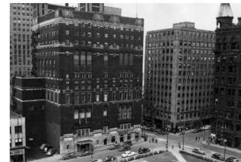
Figure 2.23 The Minnesota Building, in the middle
