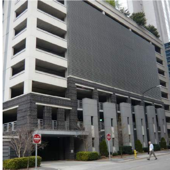
Figure 4.20 Integrate new structured parking into the development. While this structure shows appropriate screening, it is not wrapped by active uses as the design guidelines instruct.
