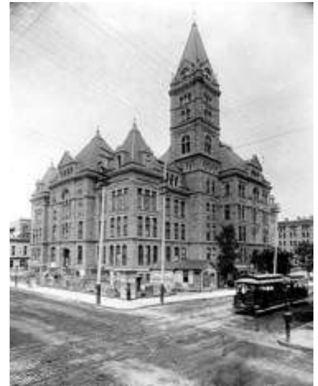
Figure 2.4 Saint Paul City Hall-Ramsey County Courthouse, ca. 1887
