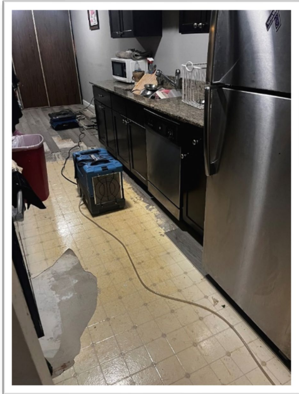
Removing presumed ACM vinyl flooring.
