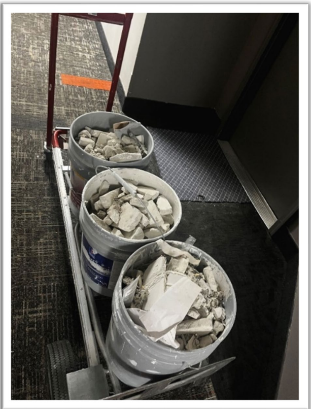
Carting uncovered suspect ACM drywall in hallways.
