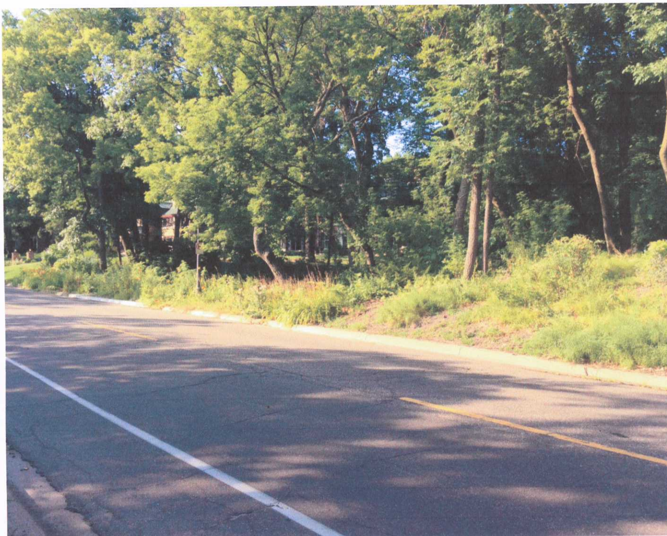
ST PAVK - EAST RIVER ROAD
