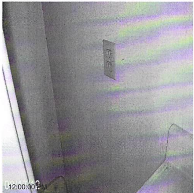
Date Completed: before: replace outlets
