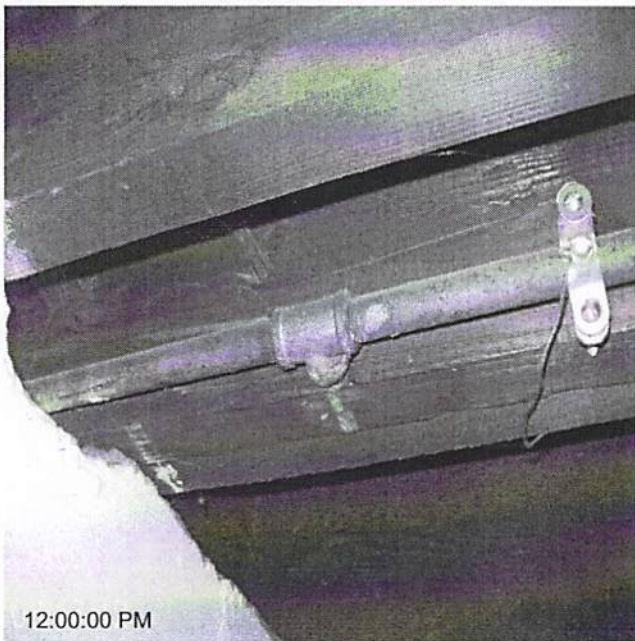
Date Completed: before: replace piping
