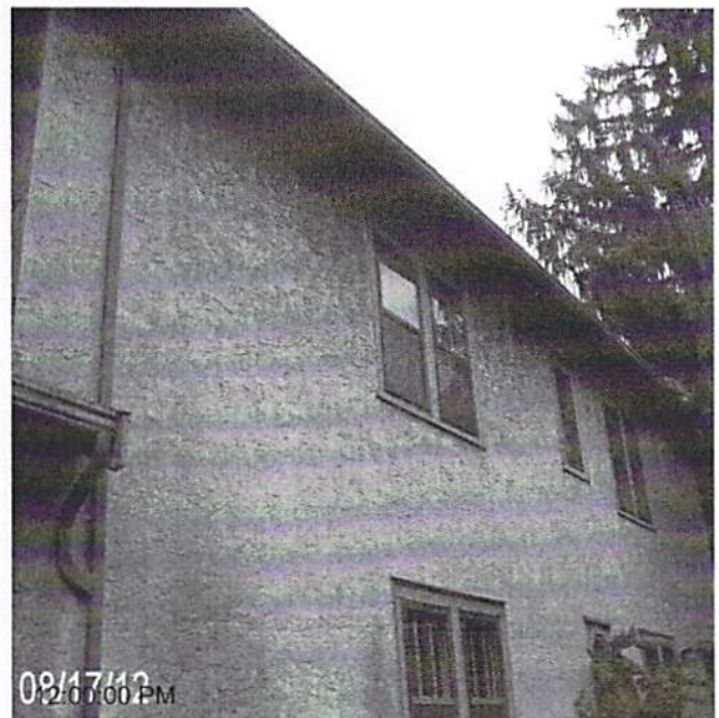
Date Completed: before: repair/pressure wash stucco
