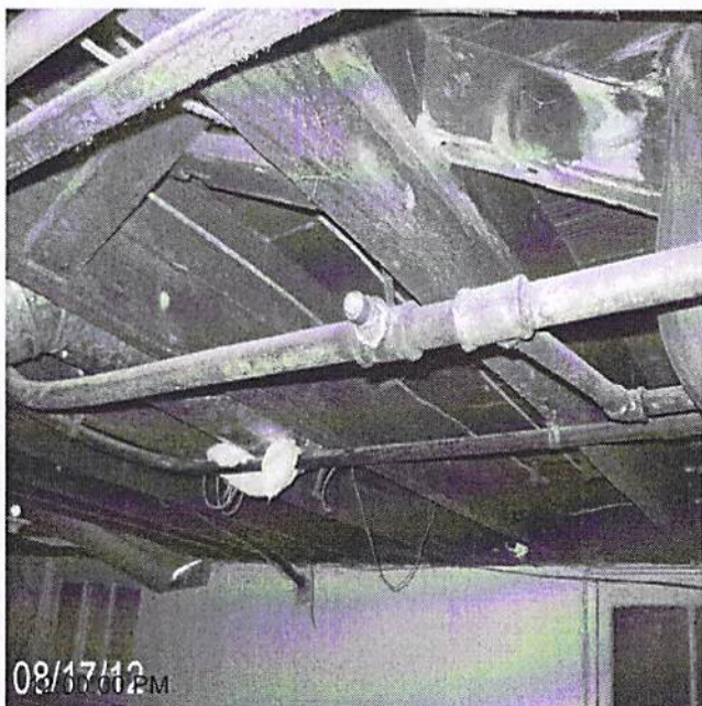
Date Completed: before: replace piping
