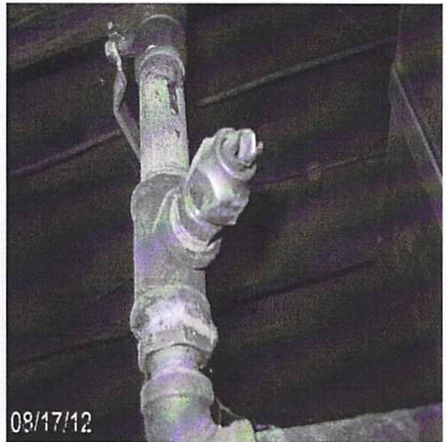
Date Completed: before: replace piping
