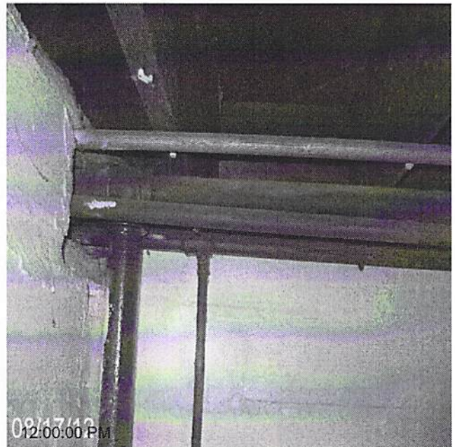
Date Completed: before: replace piping
