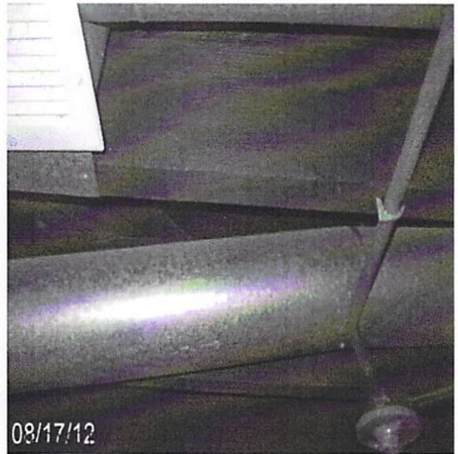
Date Completed: before: replace heating register
