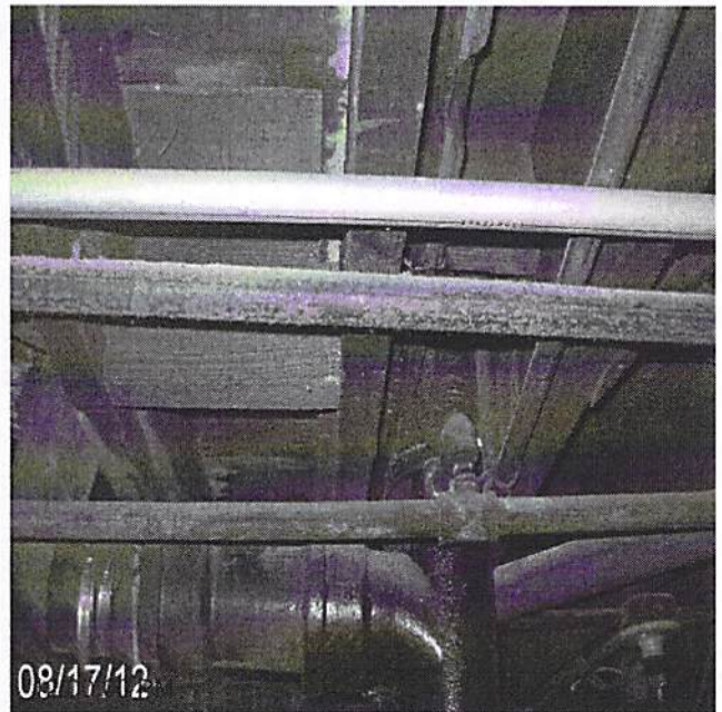
Date Completed: before: replace piping
