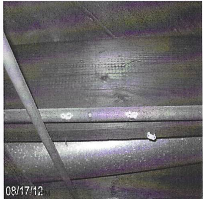
Date Completed: before: replace piping
