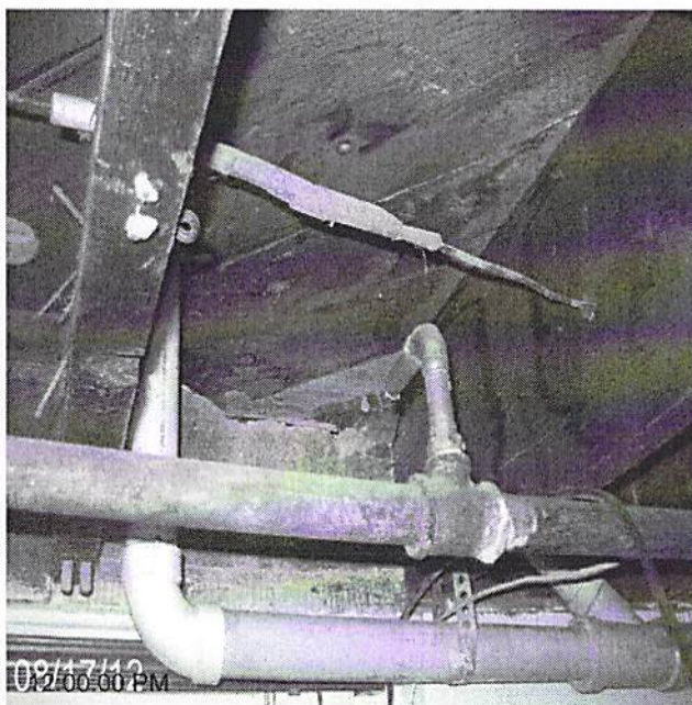
Date Completed: before: replace piping
