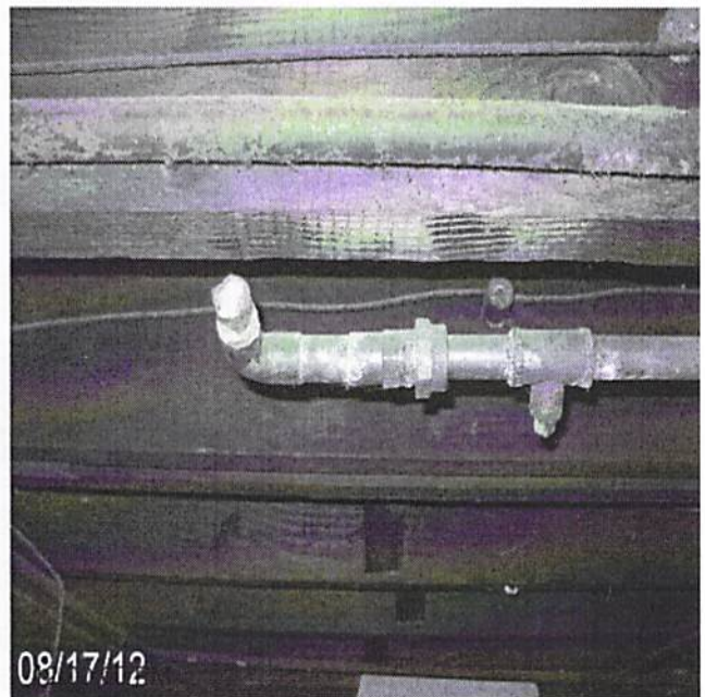
Date Completed: before: replace piping
