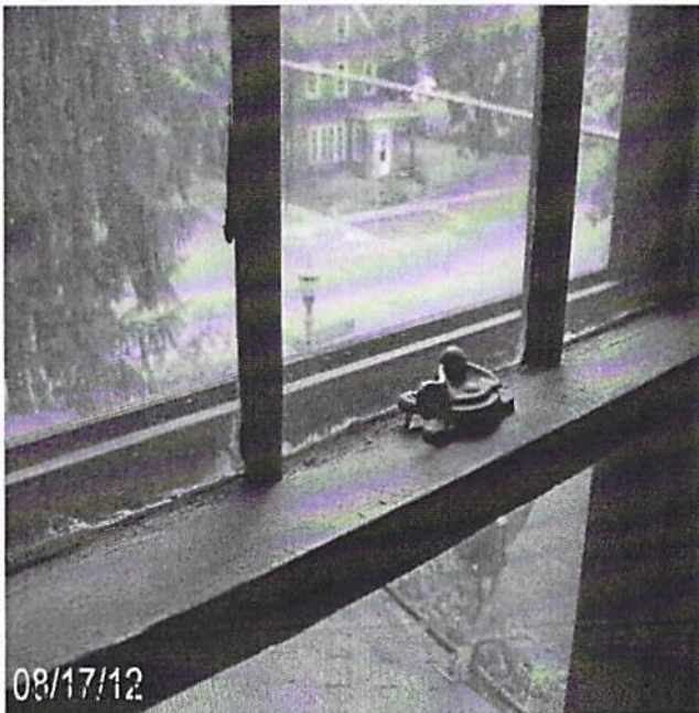
Date Completed: before: repair/replace window sash holder 1st flo
