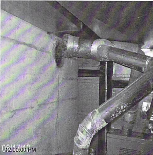
Date Completed: before: replace vent piping
