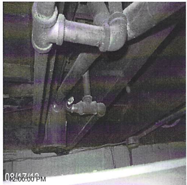
Date Completed: before: replace piping
