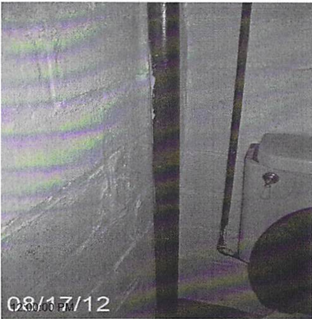
Date Completed: before: replace basement toilet
