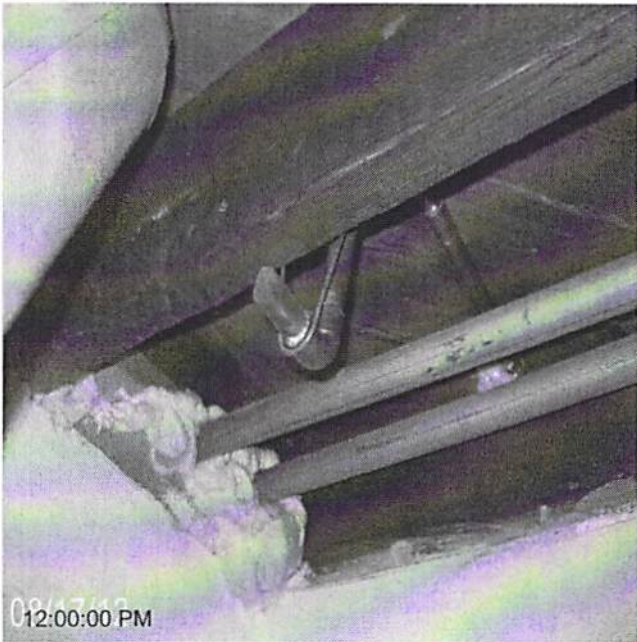
Date Completed: before: replace pipe
