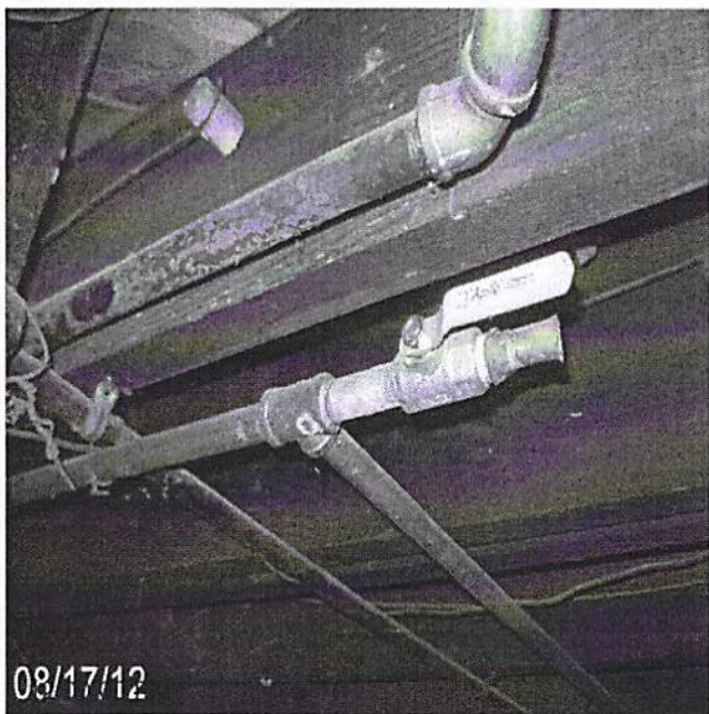
Date Completed: before: replace piping
