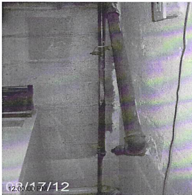
Date Completed: before: replace gas piping
