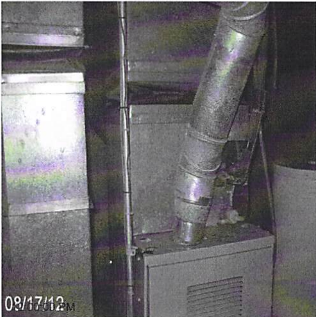
Date Completed: before: replace heating vent
