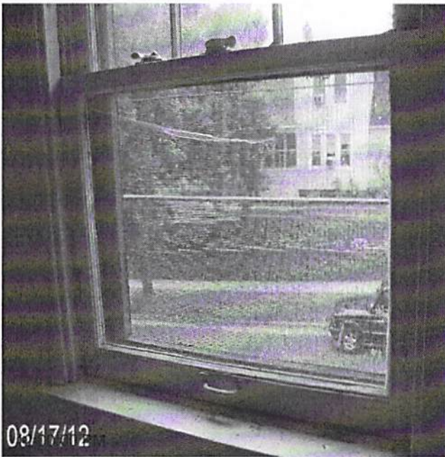
Date Completed: before: repair/replace window panes
