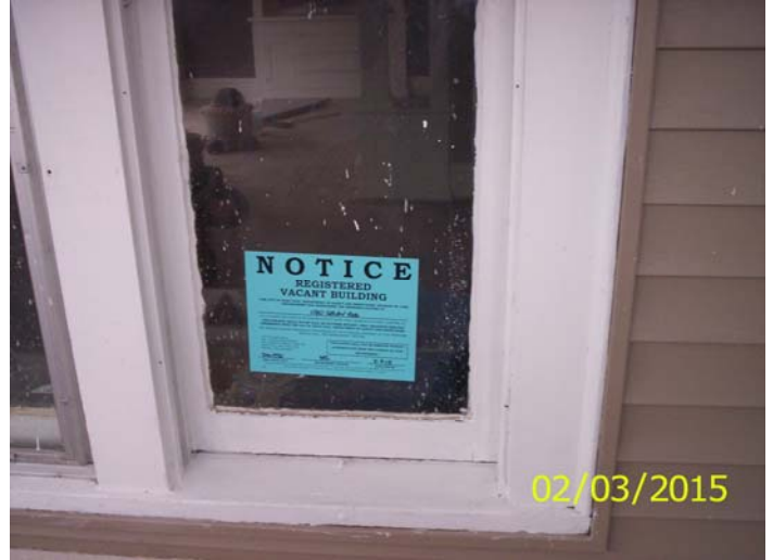
Front posting (inside porch)
