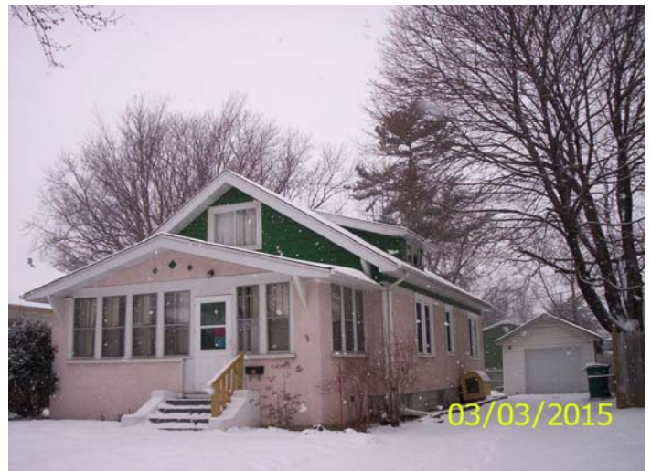
East and north sides, posting
