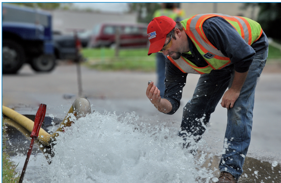
Bob Meyer gathers a water sample to test the chlorine levels and the turbidity in the water during a Uni-Directional Flush of a water hydrant in this file photo.
