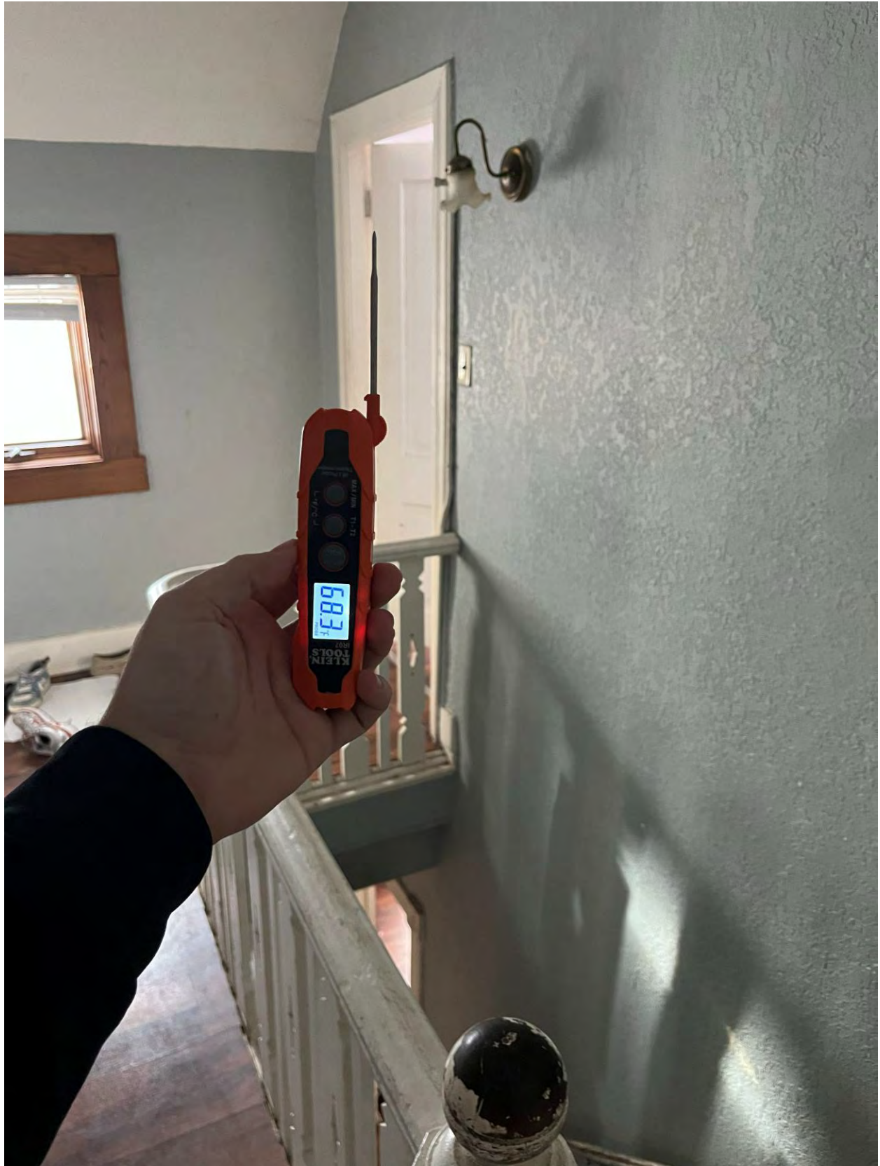
2 nd floor common area
