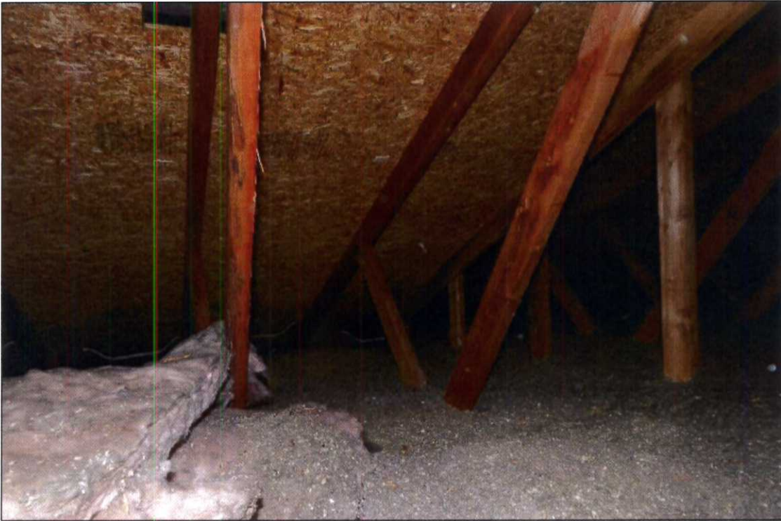
Photograph # 17: Attic above unit 203
