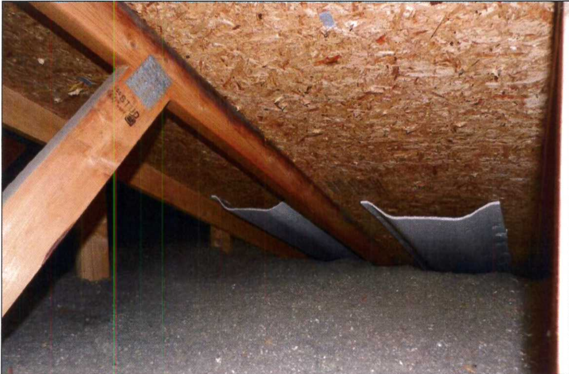
Photograph # 20: Baffles present at eaves
