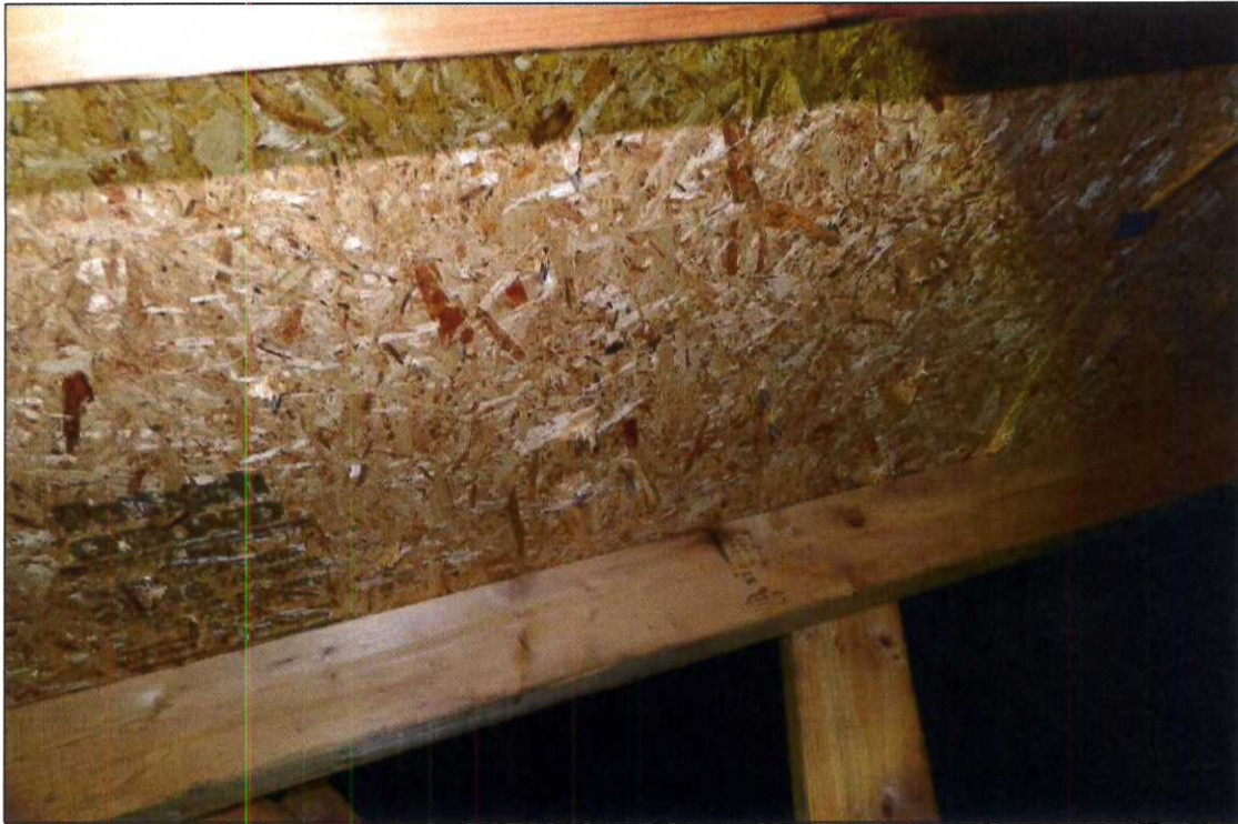
Photograph # 19: Sheathing in good condition
